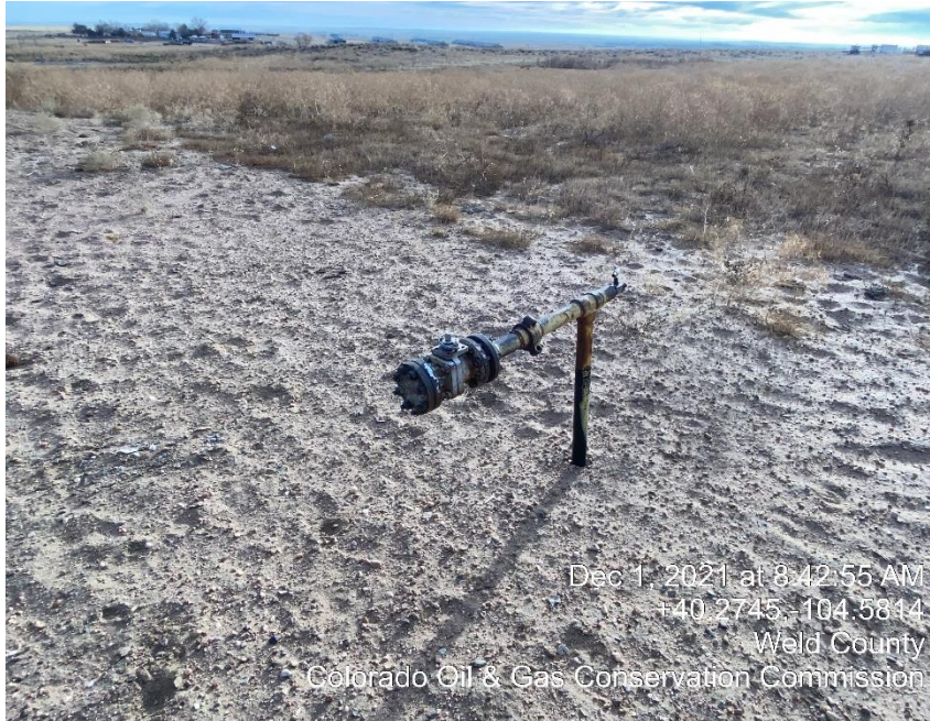
Photo #2 Unmarked riser
