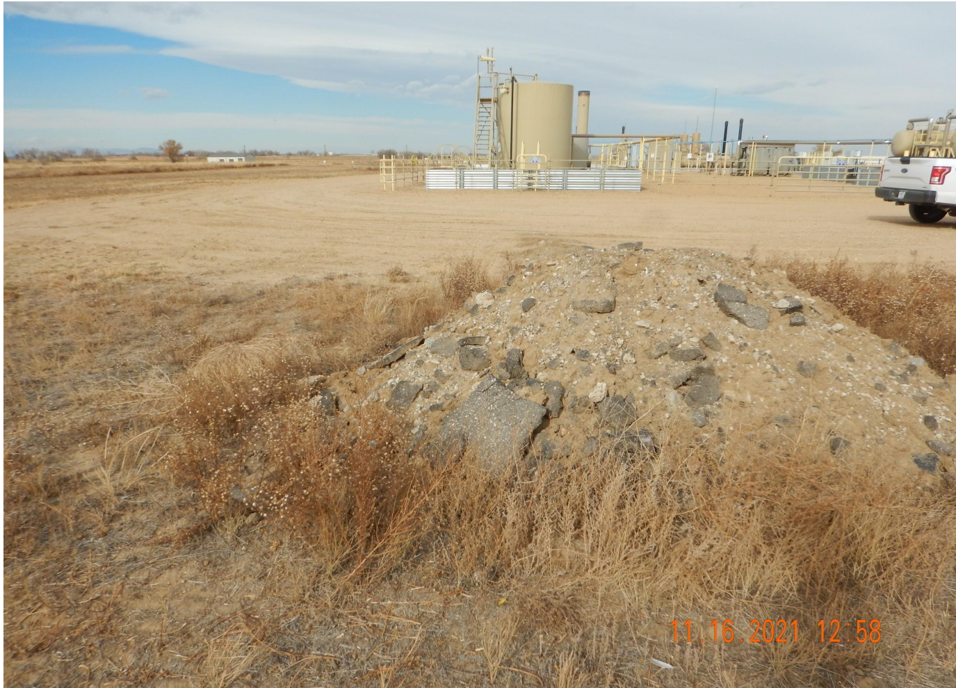
Photo 5. Photo taken from the associated offsite tank battery, facing North. The associated offsite tank battery has been removed and replaced with a new production facility for other nearby active wells. Note: A corrective action has been submitted to remove the debris pile.
