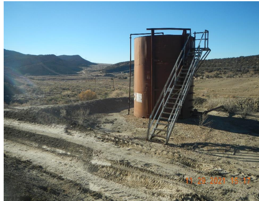
Dead weeds inside berm. Berm wall bladed over along truck access.
