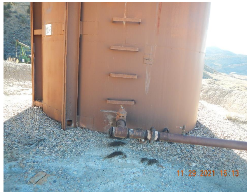
Stained soil in tank berm at flow line and load line.
