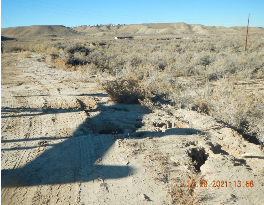
Stormwater channels on location & choking vegetation.
