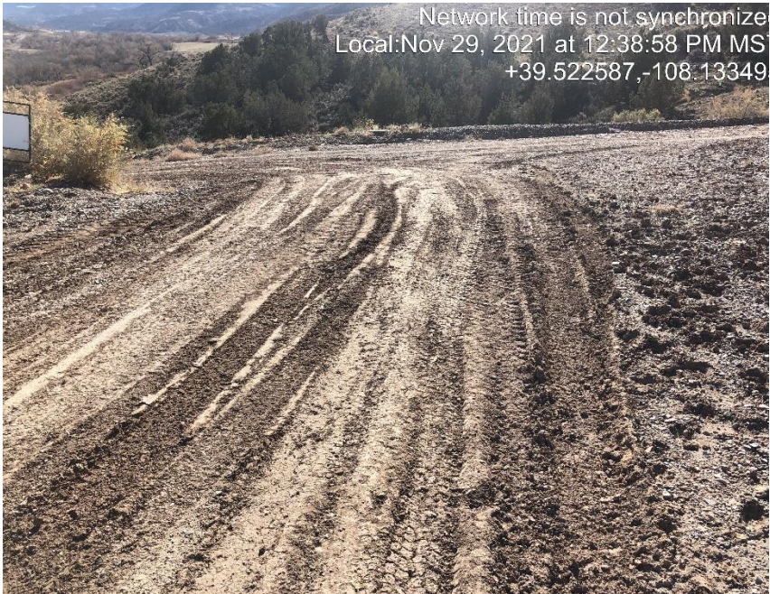
Photo #5271 No form of tracking BMP located at the entrance to location.
