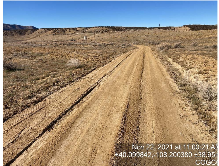
Lack of stabilization/compaction
