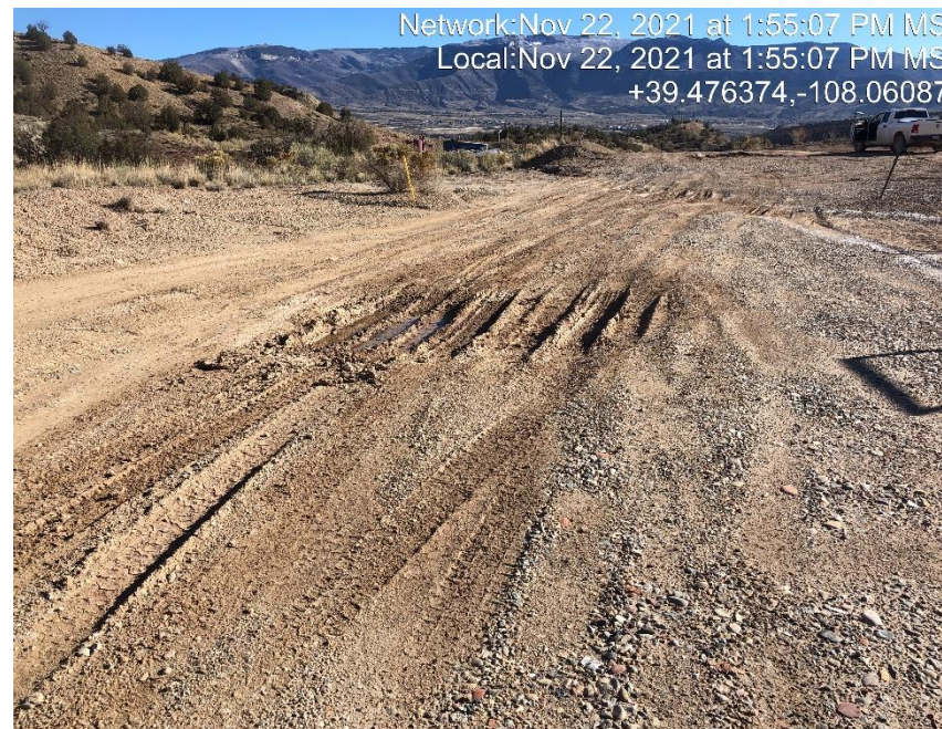
Photo #5235 Insufficient tracking BMP located at entrance to location.
