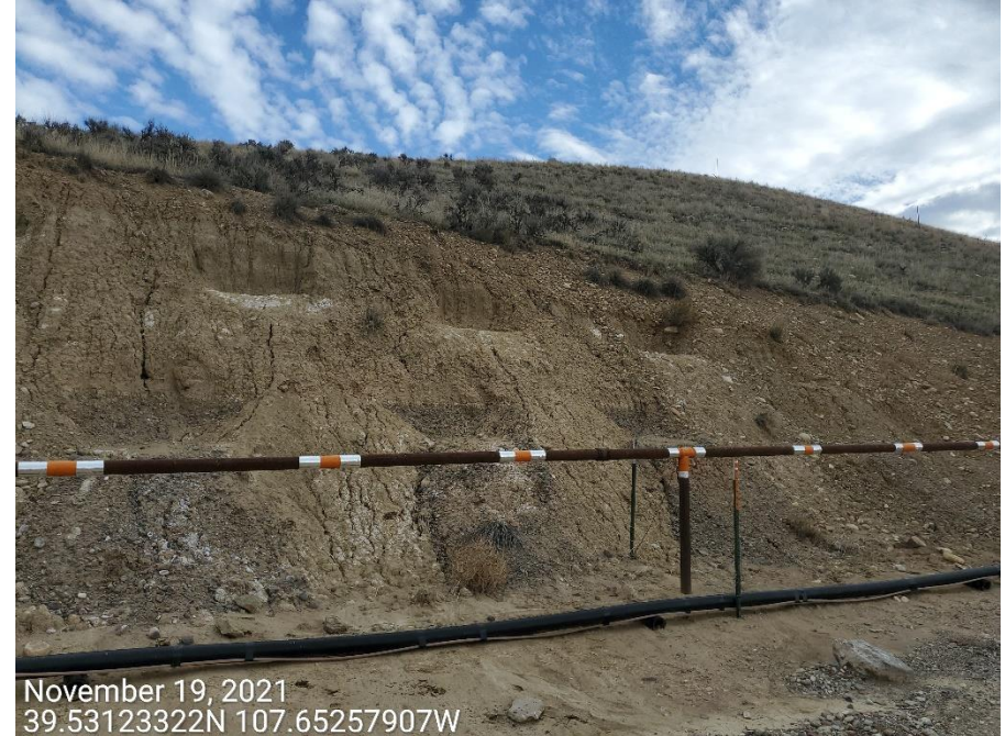
Photo 4: Photos show control measures to protect and stabilize the slopes of the Location remain missing or insufficient.
