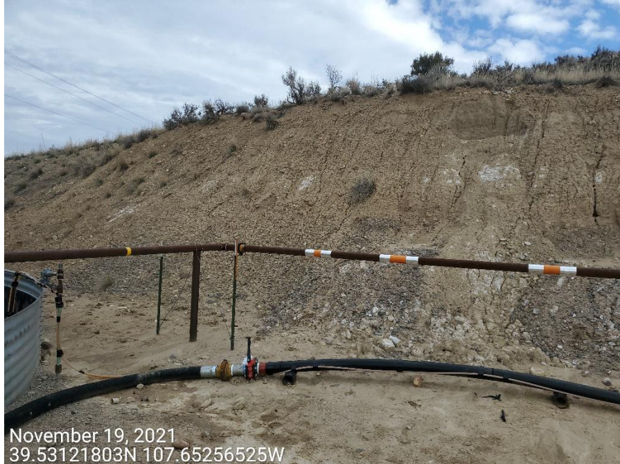
Photo 4: Photos show control measures to protect and stabilize the slopes of the Location remain missing or insufficient.
