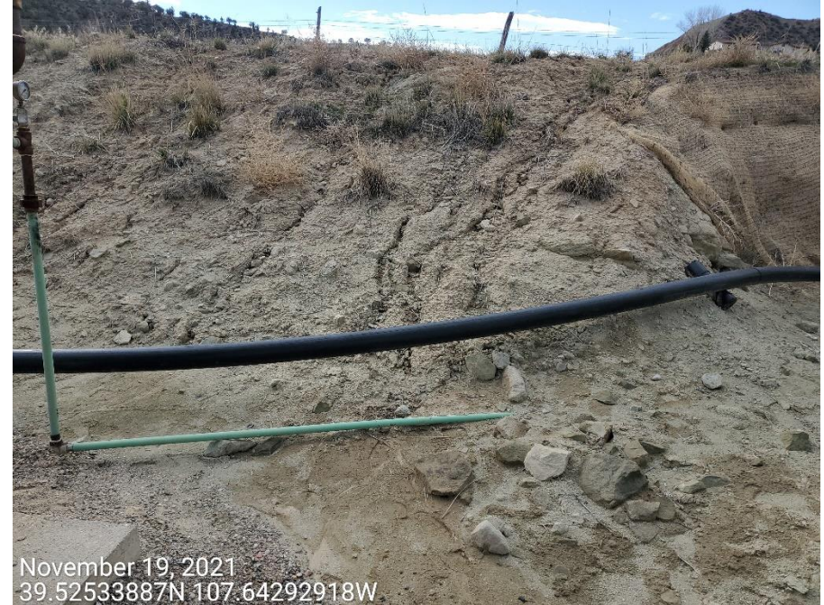
Photo 5: Photos provide examples of the cut slopes on the Location; control measures to protect and stabilize the cut slopes remains missing or insufficient per good engineering practices; erosion degradation evident. Note: yellow arrow indicating sediment deposition due to erosion at cut slopes.
