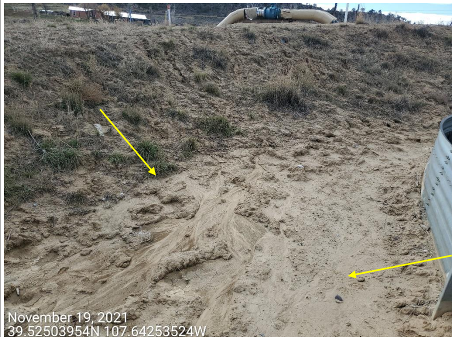
Photo 4: Photos provide examples of the cut slopes on the Location; control measures to protect and stabilize the cut slopes remains missing or insufficient per good engineering practices; erosion degradation evident. Note: yellow arrow indicating sediment deposition due to erosion at cut slopes.
