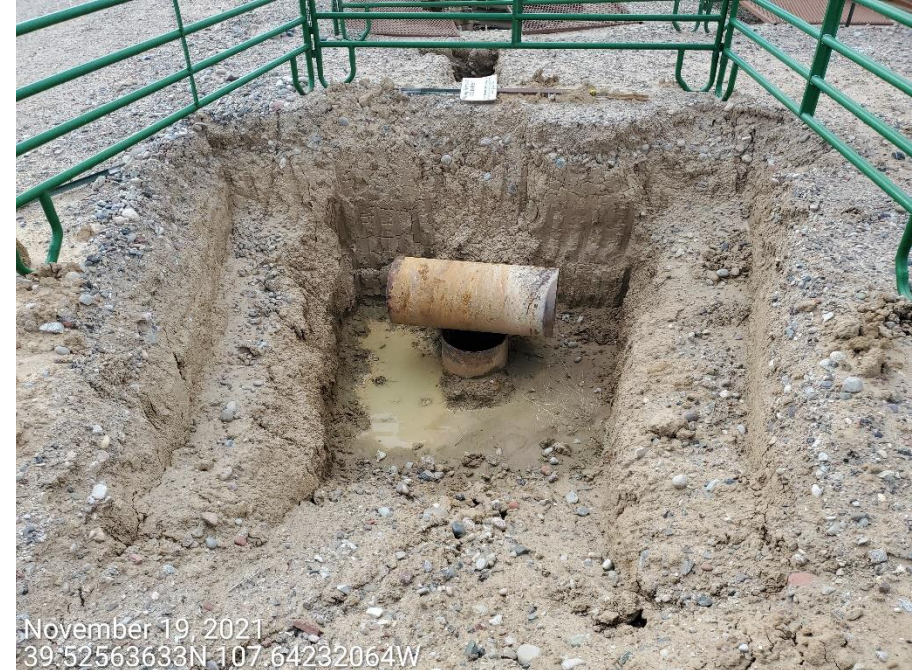
Photo 8: Photo of well API 045-18287 conductor setting; well has not been drilled; Form 2 permit expired 7/24/2020; no Form 4 to abandon well has been submitted; conductor setting requires plugging.
