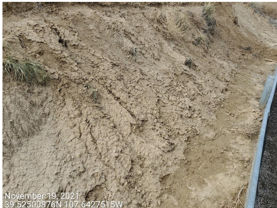
Photo 4: Photos provide examples of the cut slopes on the Location; control measures to protect and stabilize the cut slopes remains missing or insufficient per good engineering practices; erosion degradation evident. Note: yellow arrow indicating sediment deposition due to erosion at cut slopes.
