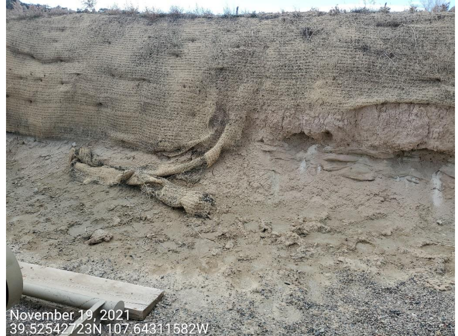
Photo 6: Photo shows erosion blankets at cut slopes behind separator equipment. Photo right shows sections of the BMP that has not been maintained in proper functioning condition.
