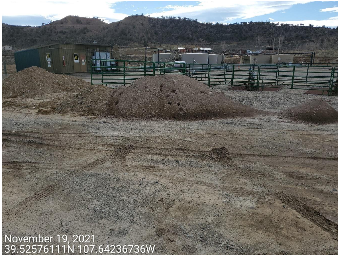
Photo 7: Photo shows stockpiled soils stored on the Location. Control measures to mitigate sediment transport from the soil stockpiles are missing or insufficient.
