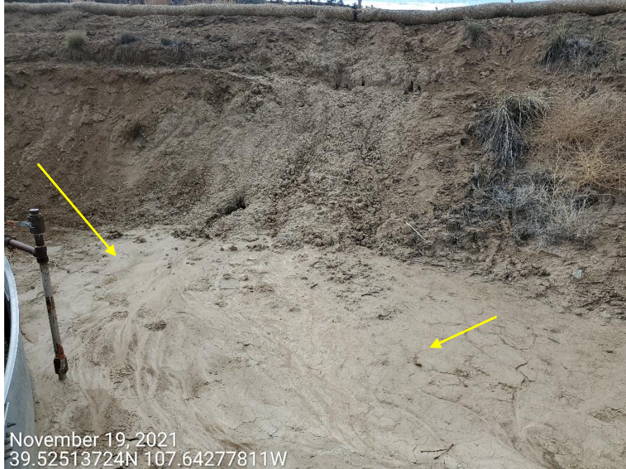
Photo 5: Photos provide examples of the cut slopes on the Location; control measures to protect and stabilize the cut slopes remains missing or insufficient per good engineering practices; erosion degradation evident. Note: yellow arrow indicating sediment deposition due to erosion at cut slopes.
