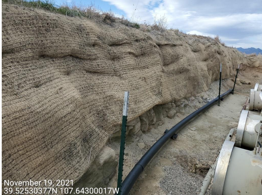
Photo 6: Photo shows erosion blankets at cut slopes behind separator equipment. Photo right shows sections of the BMP that has not been maintained in proper functioning condition.
