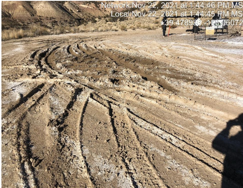
Photo #5226 Location lacks stabilization.
