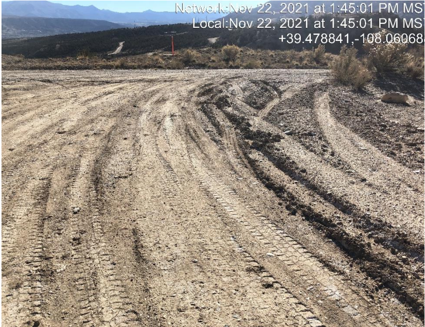
Photo #5227 Insufficient tracking BMP located at entrance to location.
