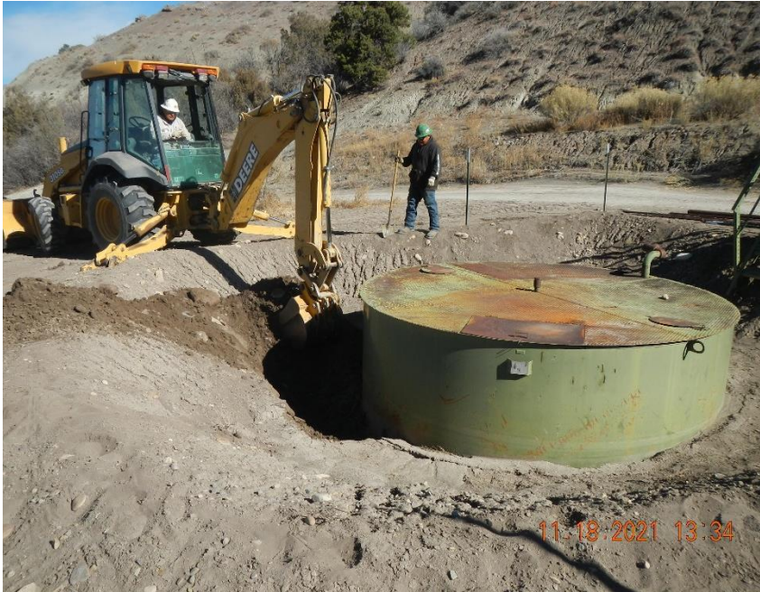
Removing soil from around the sides of the PBV.
