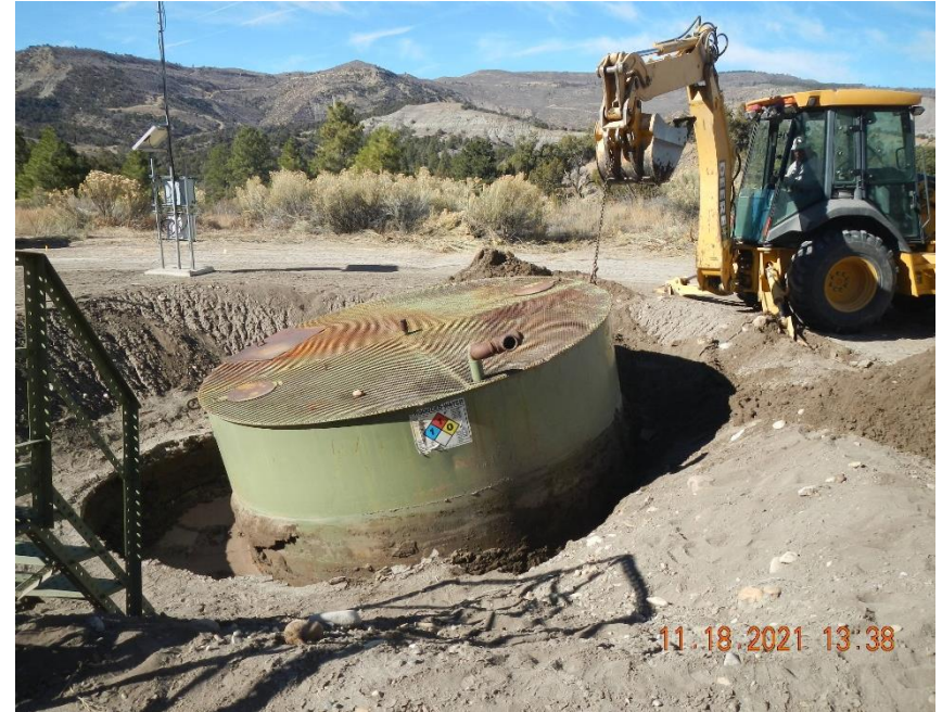
Open topped PBV being drug out of containment area.
