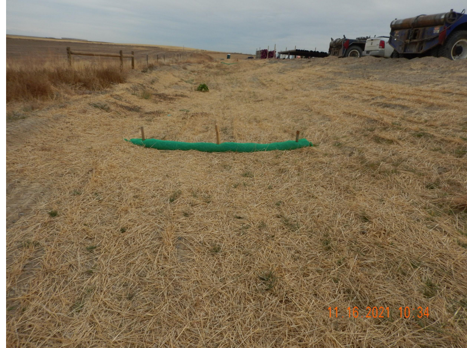
Photo 8. Photo taken from the northern location, facing East. See comments under Photo 3. Photo also illustrates the germination of desirable plant species with the fill slope and stormwater BMP area.
