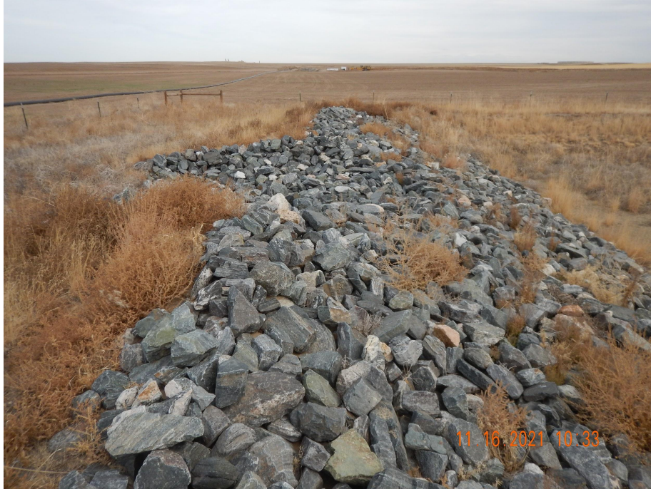
Photo 7. Photo taken from the northwestern location, facing North. Photo illustrates the stabilized outlet. There was no evidence of sediment discharge from location.
