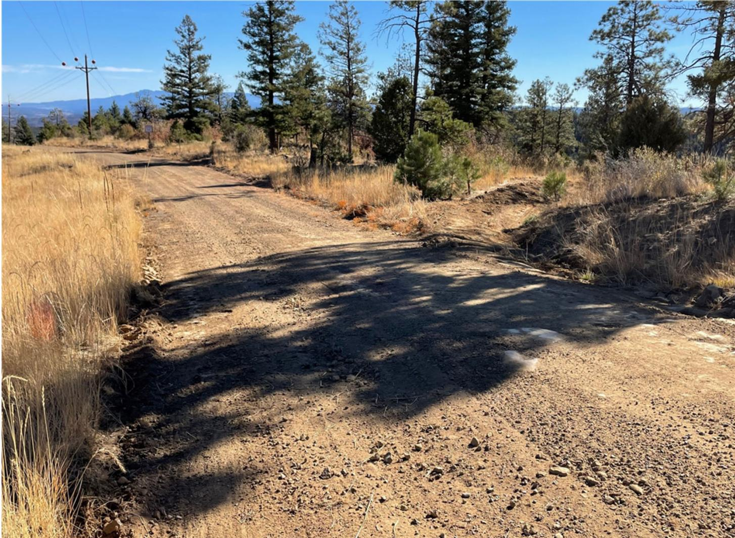
THE WATER TURNOUT WAS DOMINATED EAST OF THE WELL PAAD TO ALLOW STORMWATER TO DRAIN FROM THE ROADWAY SURFACE.
