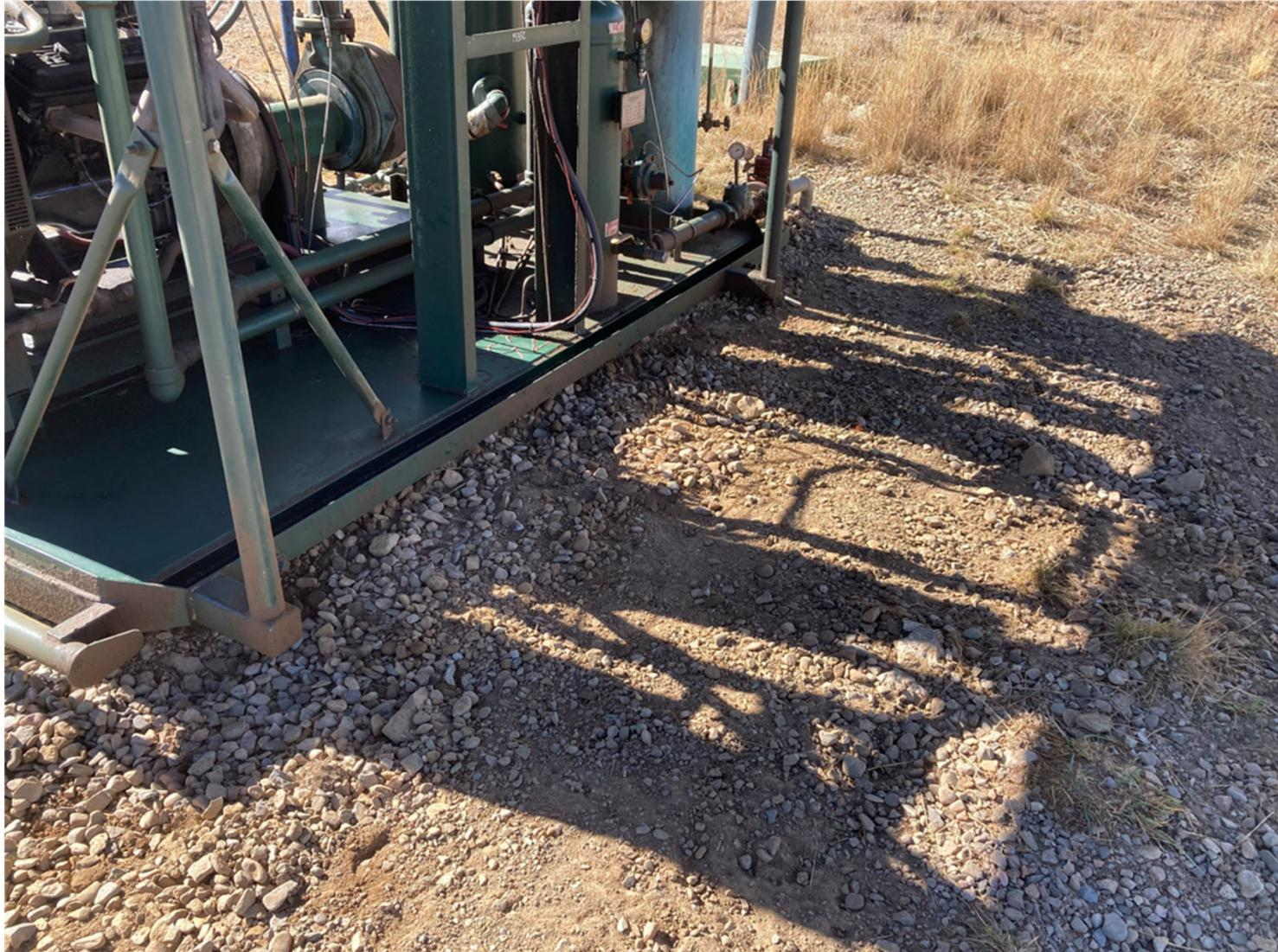
MAINTENANCE HAS BEEN PERFORMED ON THE LIQUID RING TO STOP THE OIL LEAK. THE IMPACTED SOIL NEAR THE LIQUID RING SKID WAS REMOVED FROM LOCATION.
