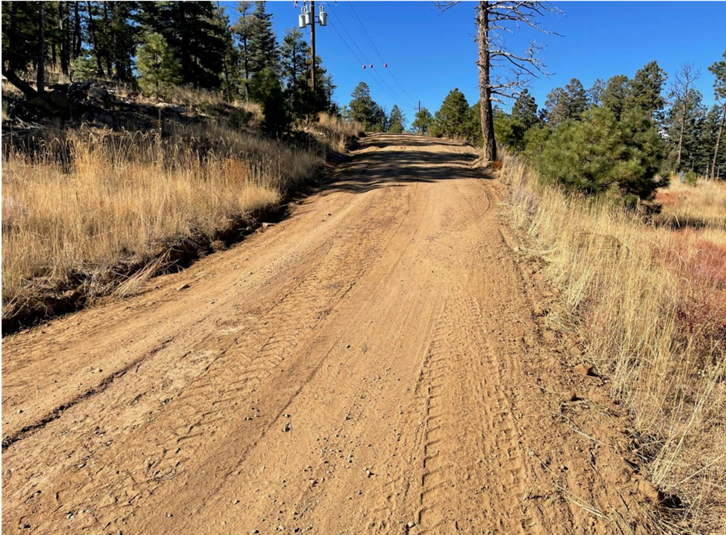
GRAVEL WAS PULLED OFF OF THE EDGE OF THE ROAD BACK ONTO THE ROAD SURFACE. GRAVEL WAS ADDED TO THE LOW AREA OF THE ROAD WHERE WATER WAS PONDING TO ALLOW STORMWATER TO DRAIN OFF OF THE ROAD SURFACE AND FOR STABILIZATION. THE LEASE ROAD WAS CROWNED TO ELIMINATE TIRE RUTS AND CREATE SHEET FLOW.
