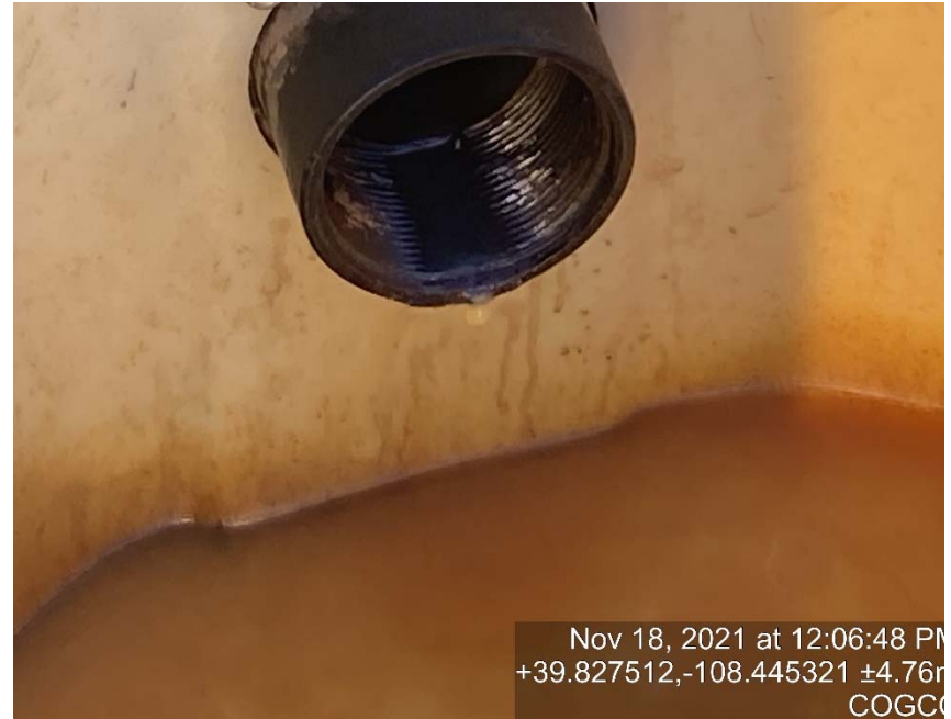
Load out lines lacking bull plugs/caps and possible slow leak
