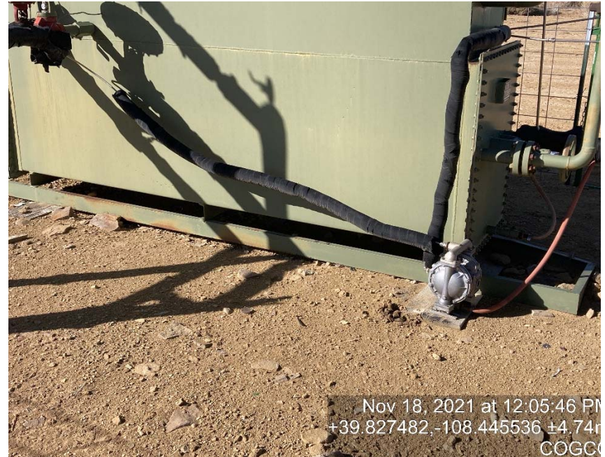
Glycol vessel lacking labeling
