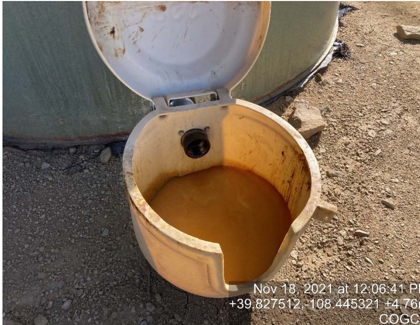
Load out lines lacking bull plugs/caps
