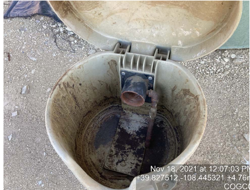
Load out lines lacking bull plugs/caps
