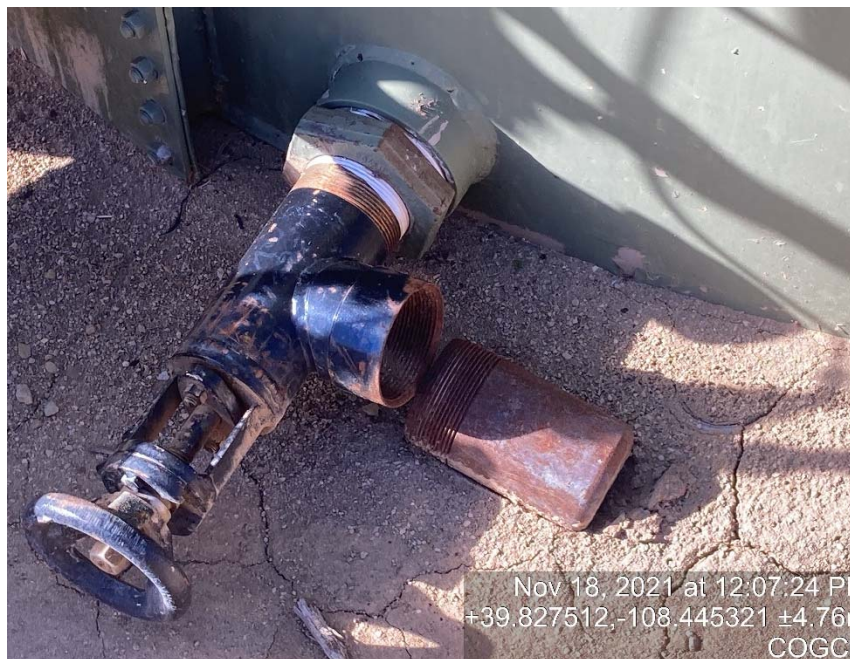
Load out lines lacking bull plugs/caps
