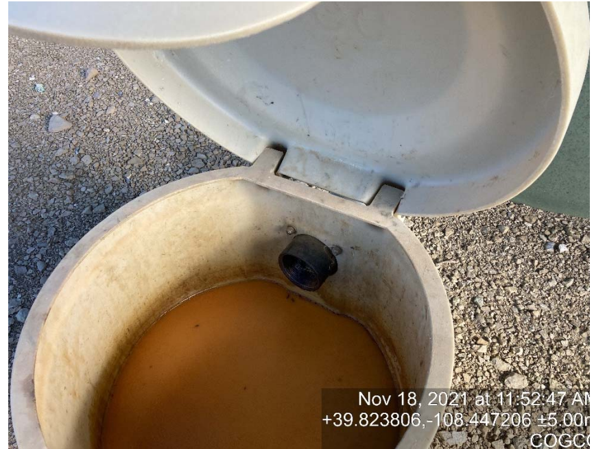
Load line missing caps/bull plugs
