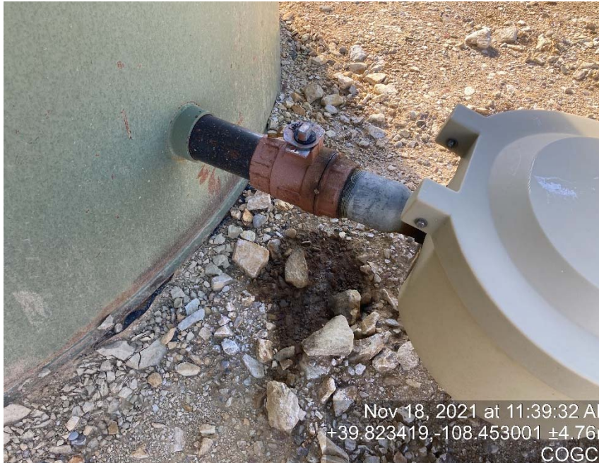
Staining under threaded ball valve/ possibly slow leak
