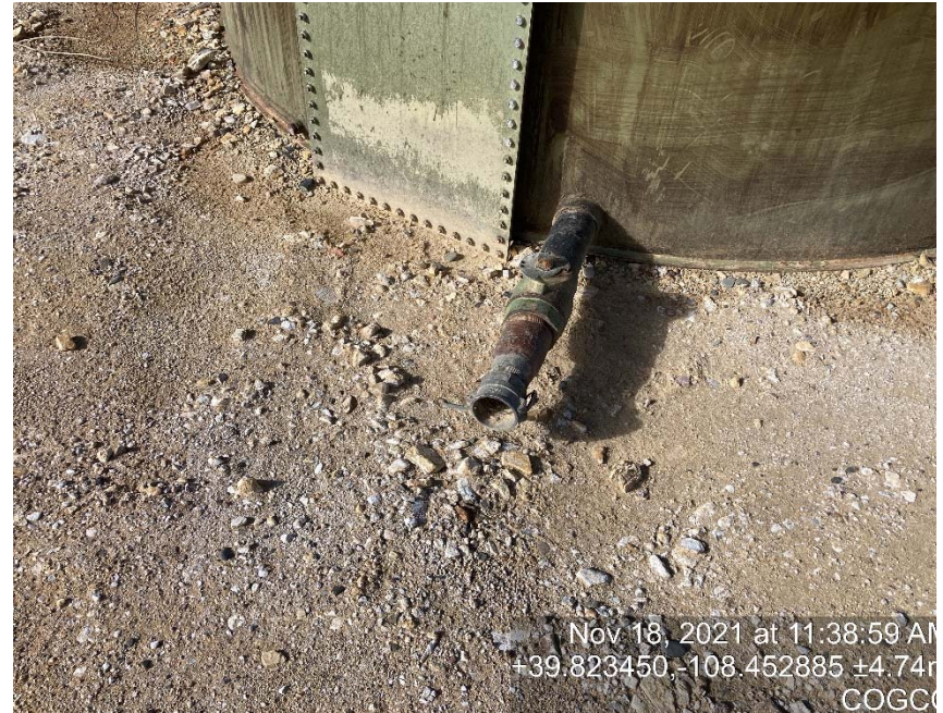
Load line missing cap/bull plug
