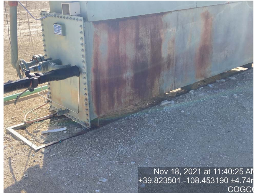
Glycol vessel lacking labeling
