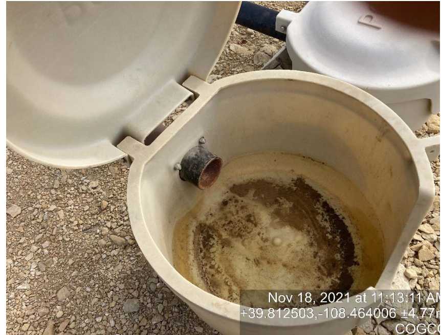
Load lines missing caps/bull plugs
