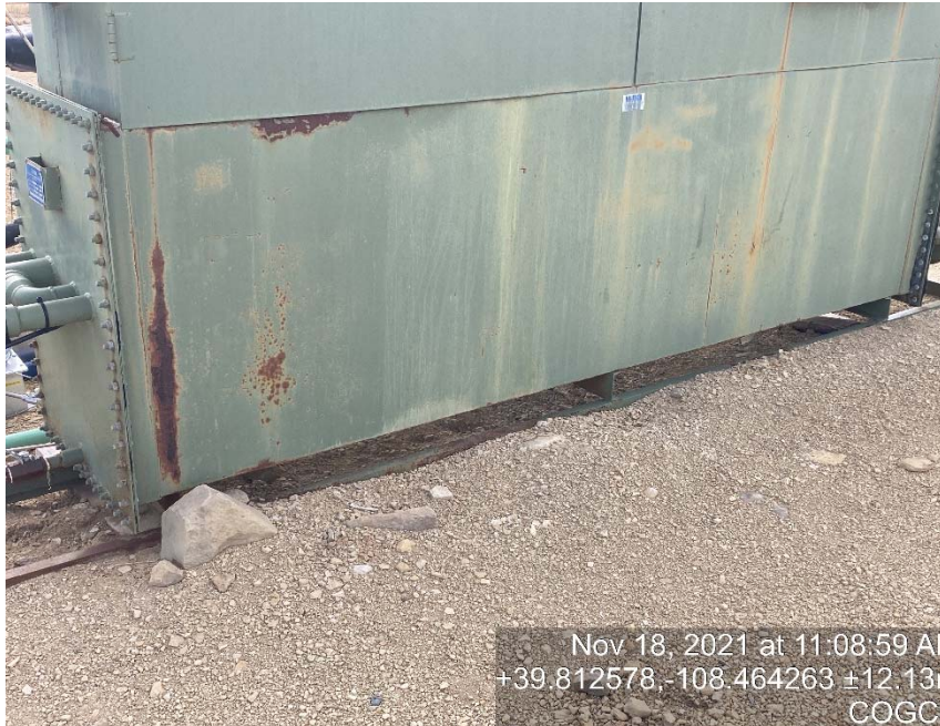
Glycol vessel lacking labeling
