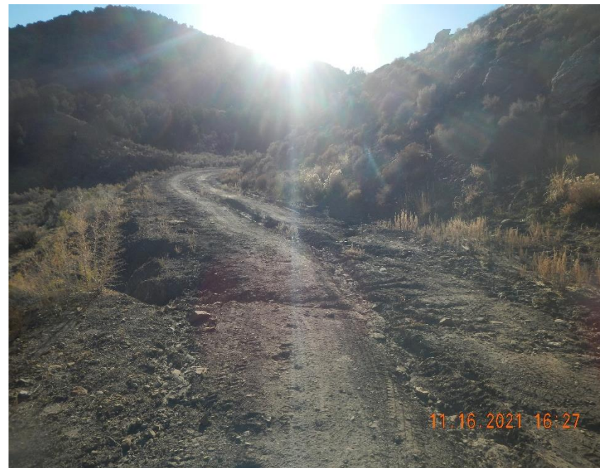
Storm water washing and riling of road.
