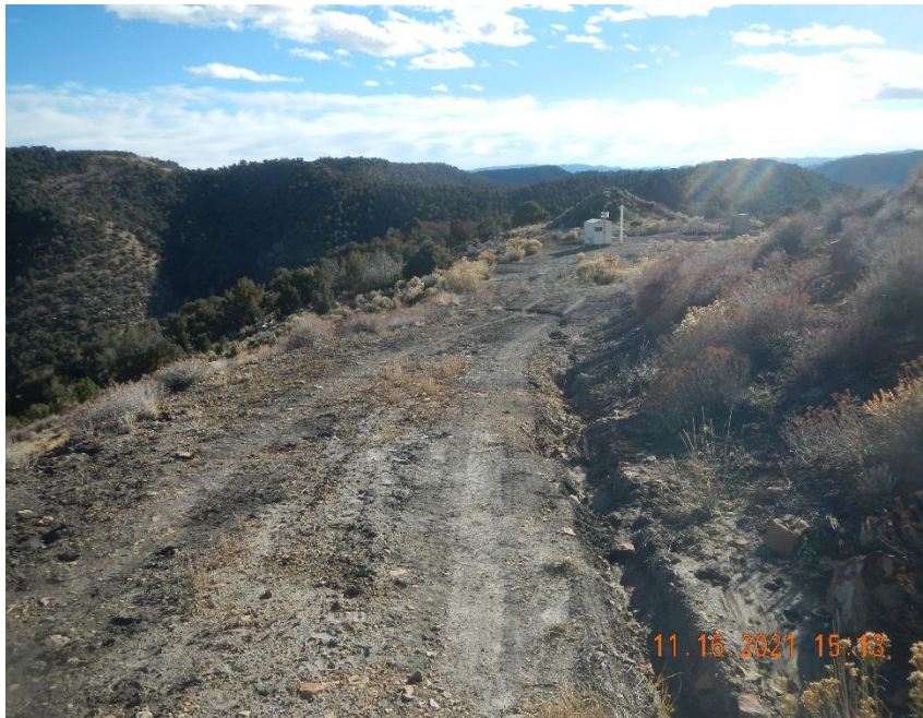
Storm water washing and riling of road.
