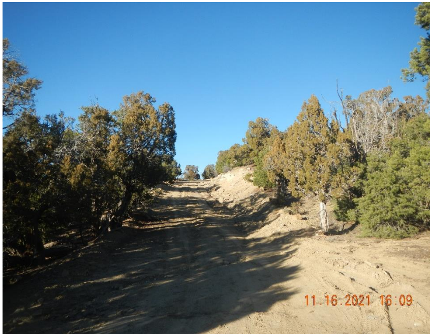
Storm water washing and riling of road.
