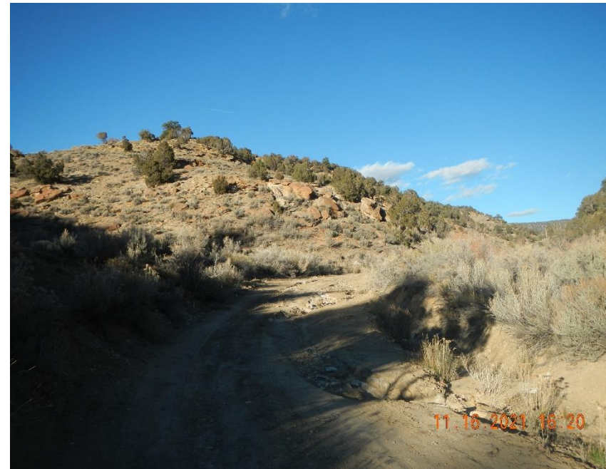
Storm water washing and riling of road.
