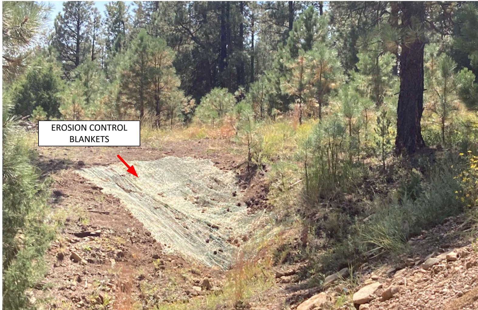
RUN OFF WAS RE-DIRECTED AWAY FROM THIS AREA. THE EROSION RILL WAS BACKFILLED. THE DISTURBED SOIL WAS SEEDED BY HAND BROADCAST WITH AN APPROVED CPW SEED MIX TO ESTABLISH VEGETATION. EROSION CONTROL BLANKETS WERE INSTALLED FOR SOIL STABILIZATION AND EROSION CONTROL.
