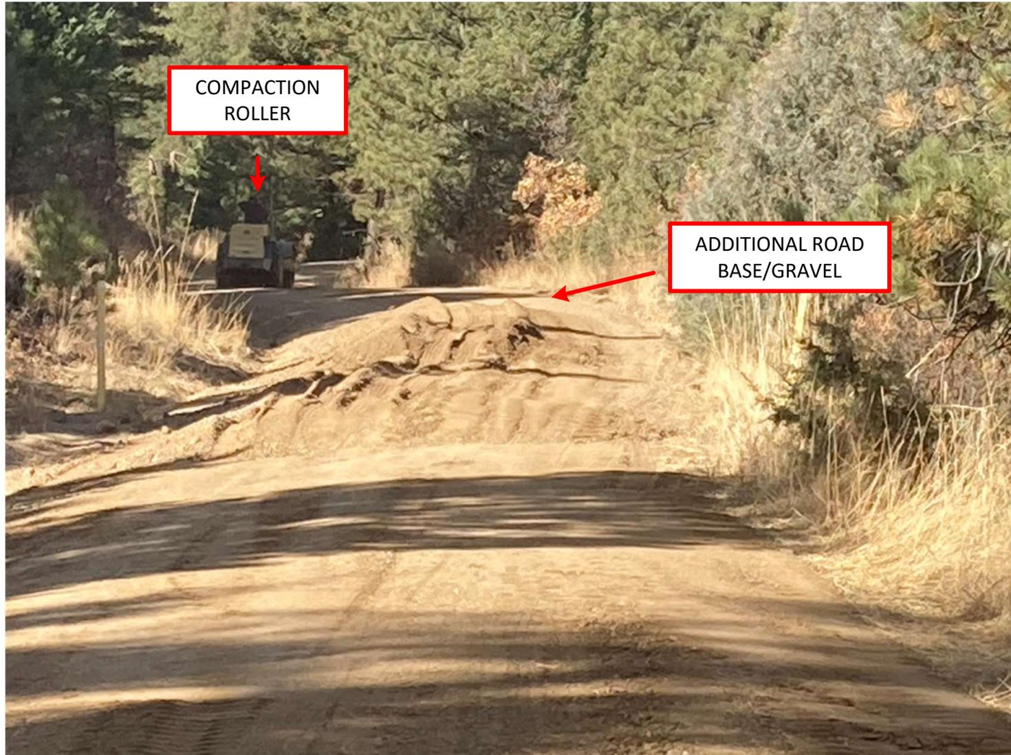
THE ROAD SURFACE WAS CROWNED TO CREATE SHEET FLOW AND ELIMINATE THE TIRE RUTS. ADDITIONAL ROAD BASE/GRAVEL WAS INSTALLED TO THE ROADWAY SURFACE TO PROVIDE STABILIZATION. A COMPACTION ROLLER WAS USED DURING THE INSTALLATION TO COMPACTED THE ROAD BASE.
