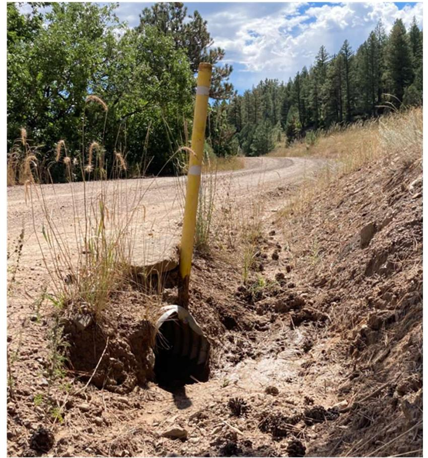
THE SEDIMENT ACCUMULATION IN THE CULVERT INLETS ALONG BIG BINGHAM CANYON WERE REMOVED.
