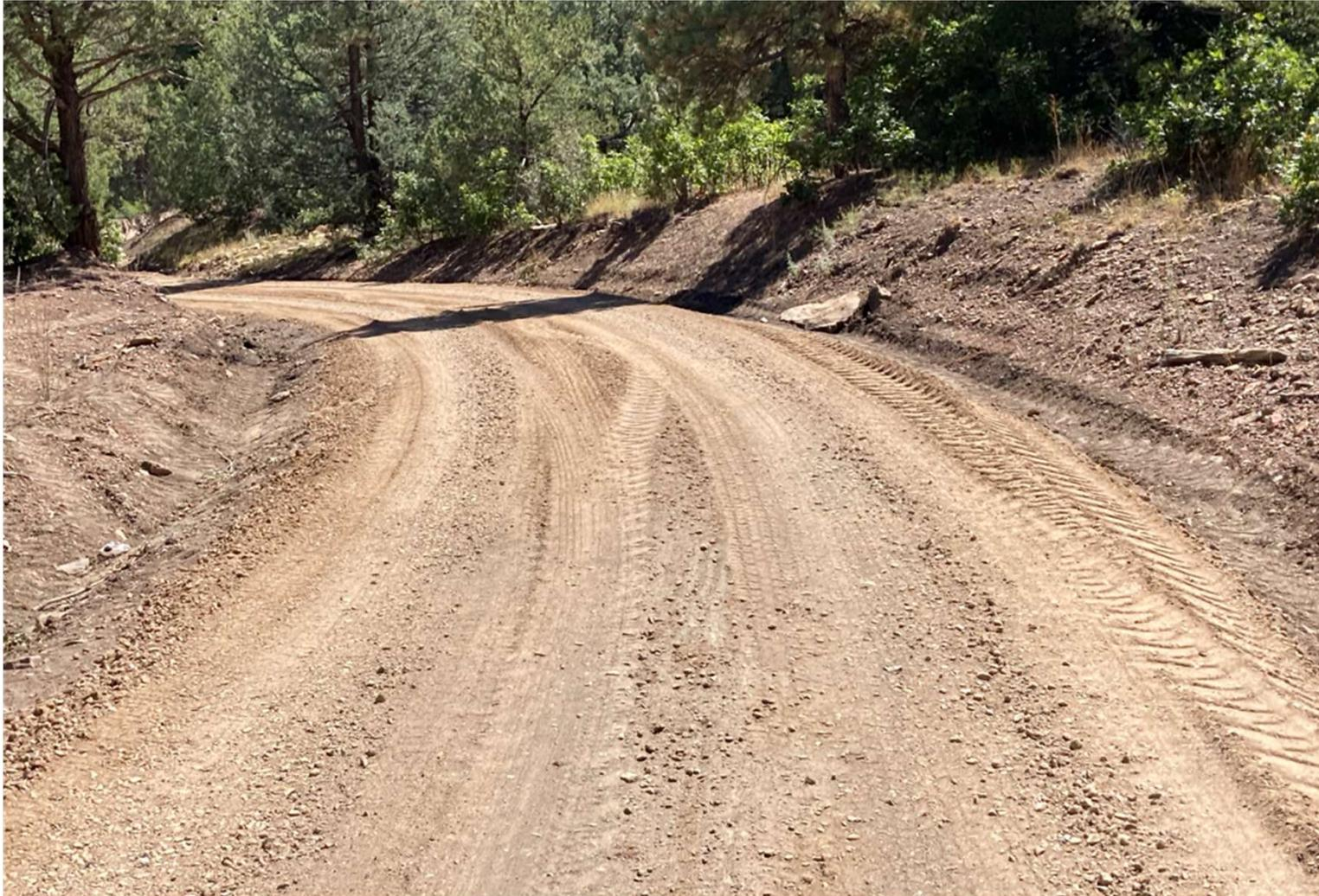
THE ROAD SURFACE WAS CROWNED TO CREATE SHEET FLOW AND ELIMINATE THE TIRE RUTS. ADDITIONAL ROAD
