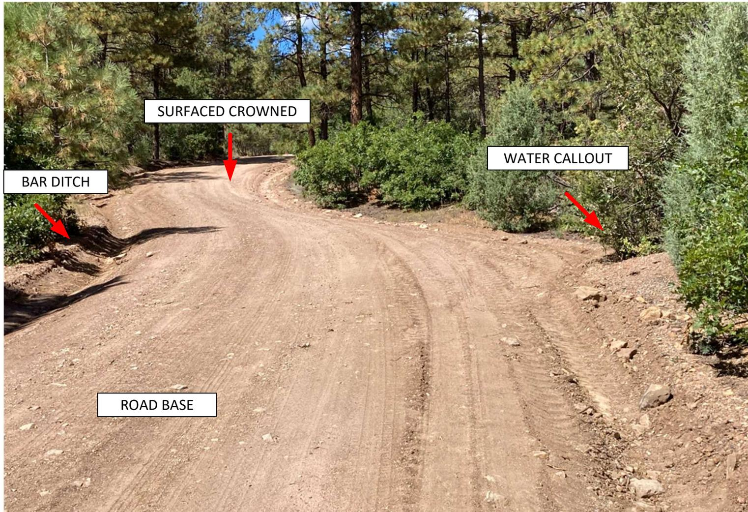
WATER CALLOUTS WERE INSTALLED TO MOVE STORMWATER AWAY FROM THE LEASE ROAD. THE ROAD SURFACE WAS CROWNED TO CREATE SHEET FLOW AND ELIMINATE THE TIRE RUTS. ADDITIONAL ROAD BASE/GRAVEL WAS INSTALLED TO THE ROADWAY SURFACE TO PROVIDE ADDED STABILIZATION.
