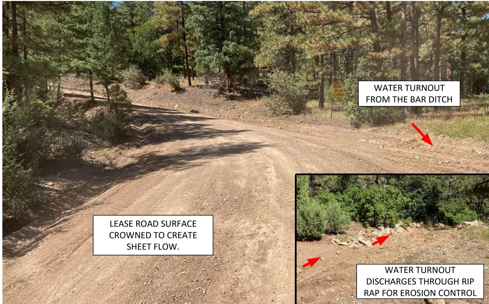
THE BLUE PIPE FRAGMENTS WERE PICKED UP AND DISPOSED OF. THE EXISTING WATER CALLOUT WAS DOMINATED TO PROVIDE POSITIVE FLOW OF STORMWATER OFF OF THE LEASE ROAD. THE FLOW FROM THE WATER TURNOUT INTERCEPTS RIP RAP FOR EROSION CONTROL DURING DISCHARGE. THE ROAD SURFACE WAS CROWNED TO CREATE SHEET FLOW AND ELIMINATE THE TIRE RUTS. ADDITIONAL ROAD BASE/GRAVEL WAS INSTALLED TO THE ROADWAY SURFACE TO PROVIDE ADDED STABILIZATION.
