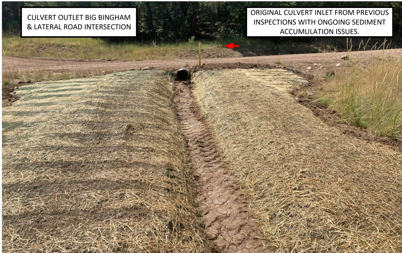
THE CULVERT OUTLET ON THE MAIN LEASE ROAD WAS BELOW GRADE AND WOULD NOT DRAIN PROPERLY. DRAINAGE WAS ESTABLISHED FOR THE OUTLET AND THE DISTURBED SOIL WAS SEEDED USING THE CPW APPROVED SEED MIX TO PROMOTE THE ESTABLISHMENT OF VEGETATION. EROSION CONTROL BLANKETS WERE INSTALLED FOR TEMPORARY SOIL STABILIZATION.
