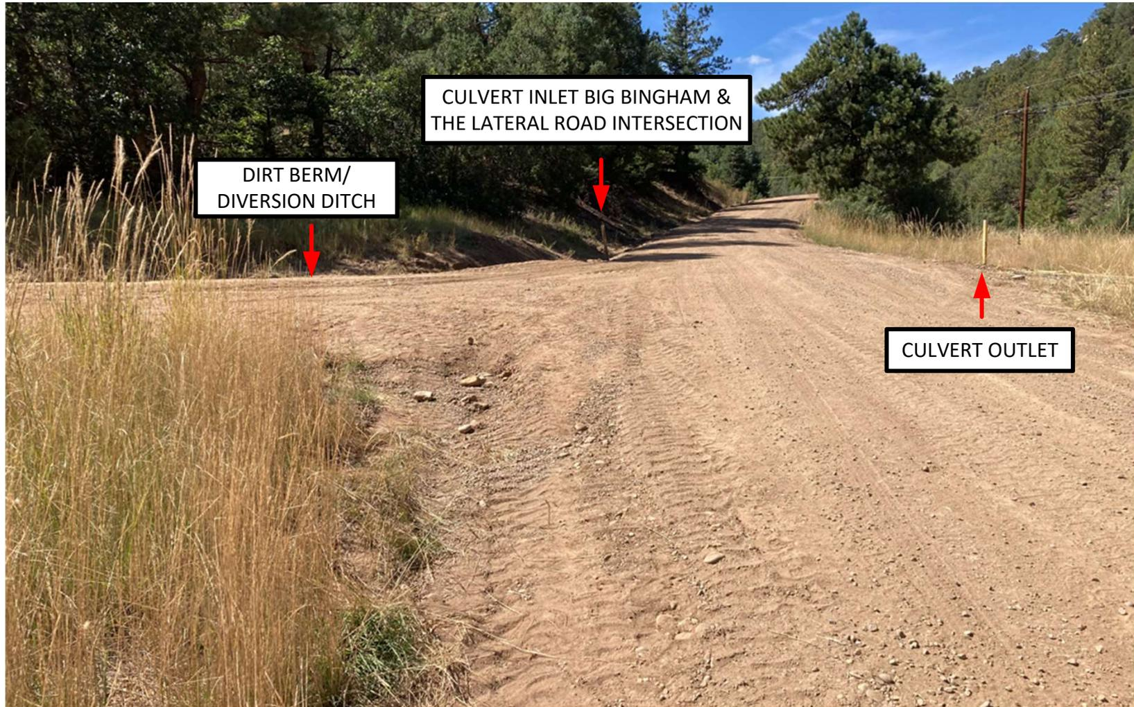
THE ROAD SURFACE WAS REGRADED TO CREATE SHEET FLOW AND ELIMINATE THE SURFACE EROSION. THE DIRT BERM/ DIVERSION DITCH WAS DOMINATED TO DIRECT RUN OFF FROM THE UPGRADIENT LATERAL ROAD TO THE CULVERT INLET ON THE MAIN ROAD. THE SEDIMENT ACCUMULATION WAS REMOVED FROM THE CULVERT INLET AND POSITIVE DRAINAGE WAS ESTABLISHED FOR THE CULVERT OUTLET.
