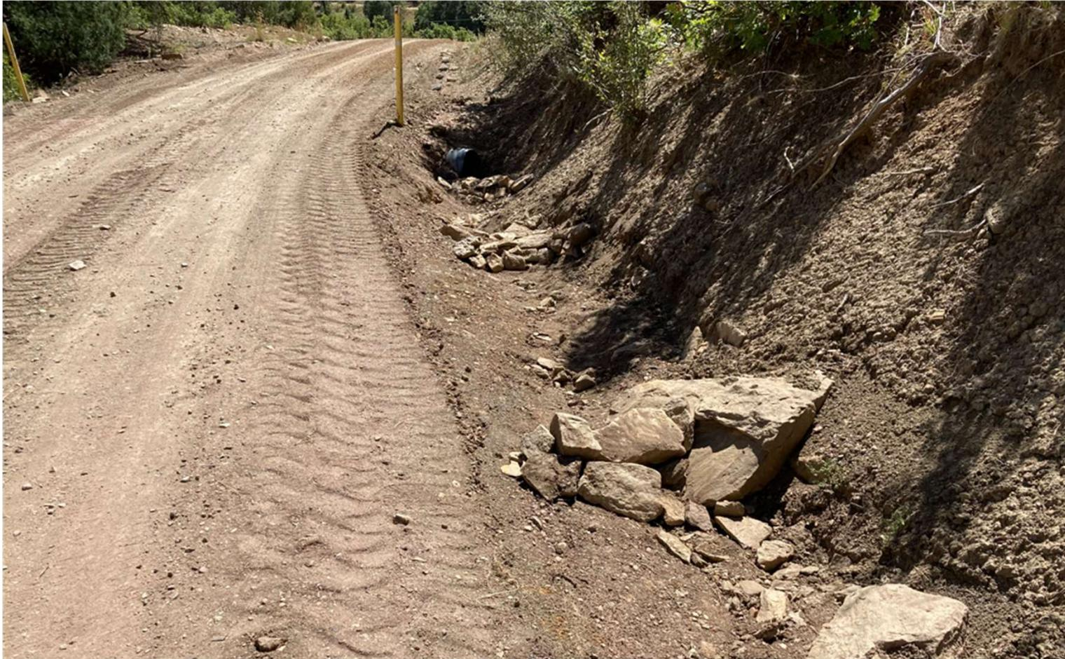
ROCK CHECKS DAMS WERE PLACED IN THE BAR DITCH UP GRADIENT OF THE CULVERT INLET TO ABSORB ENERGY AND PROVIDE SEDIMENT FILTRATION FROM RUN OFF. THE ROAD SURFACE WAS CROWNED TO CREATE SHEET FLOW AND ELIMINATE THE TIRE RUTS. ADDITIONAL ROAD BASE WAS INSTALLED TO THE ROAD SURFACE TO PROVIDE ADDED STABILIZATION.
