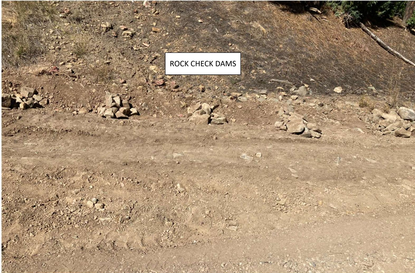
ROCK CHECKS DAMS WERE PLACED IN THE BAR DITCH TO DISSIPATE ENERGY AND PROVIDE SEDIMENT FILTRATION DURING RUN OFF EVENTS.
