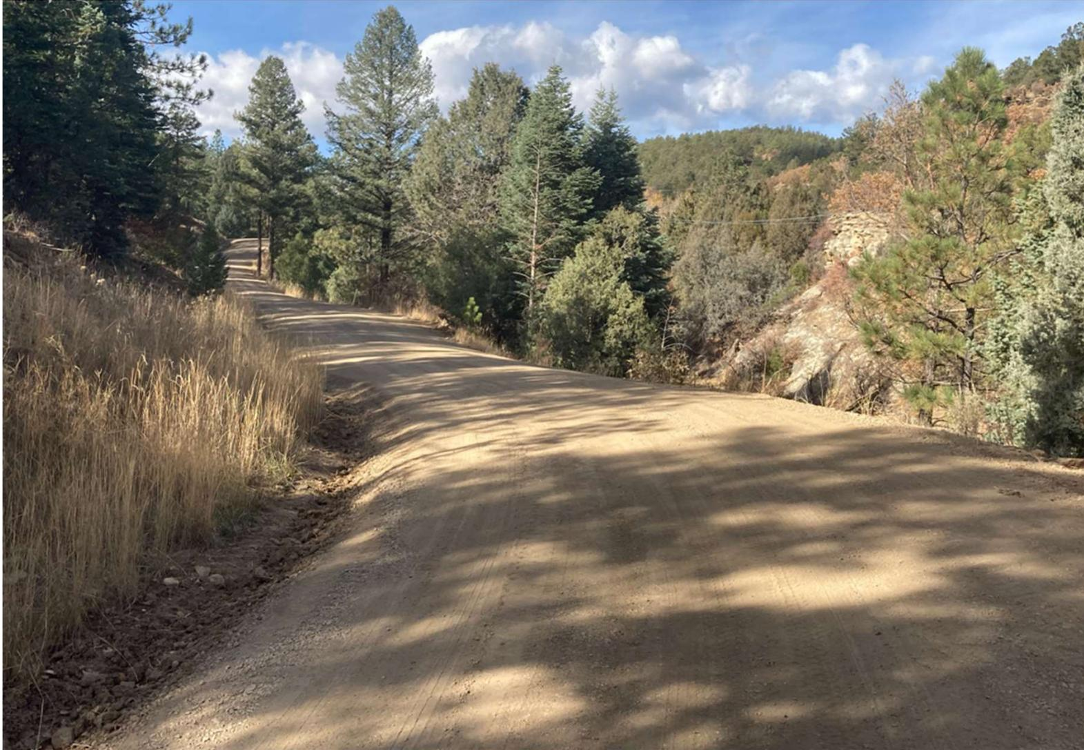
THE ROAD SURFACE WAS CROWNED TO CREATE SHEET FLOW AND ELIMINATE THE TIRE RUTS. ADDITIONAL ROAD BASE/
