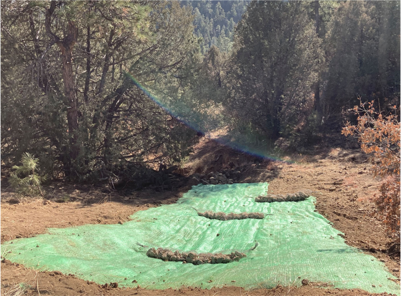
THE EROSION RILL ON THE FILL SLOPE WAS REPAIRED. TURF REINFORCEMENT MATS, ROCK SOCKS AND ARMOR WAS INSTALLED IN THE FLOWLINE FOR EROSION CONTROL.
