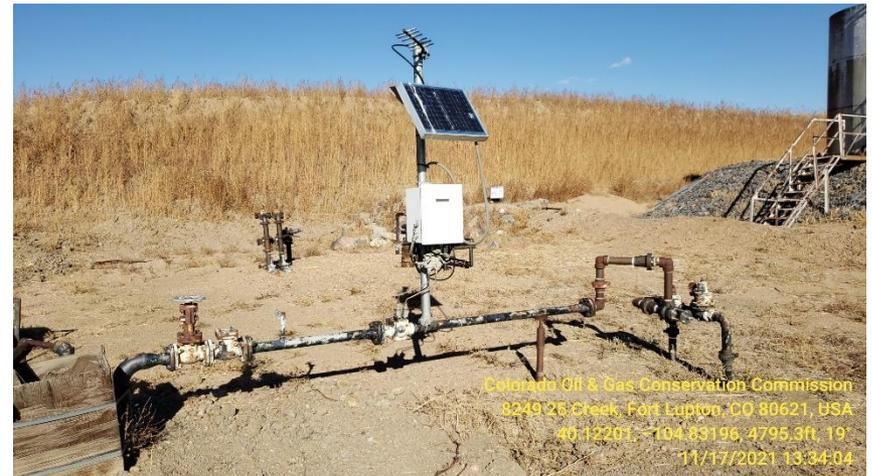
Photo 8 Gas meter run, card in box indicates that calibration is not current.
