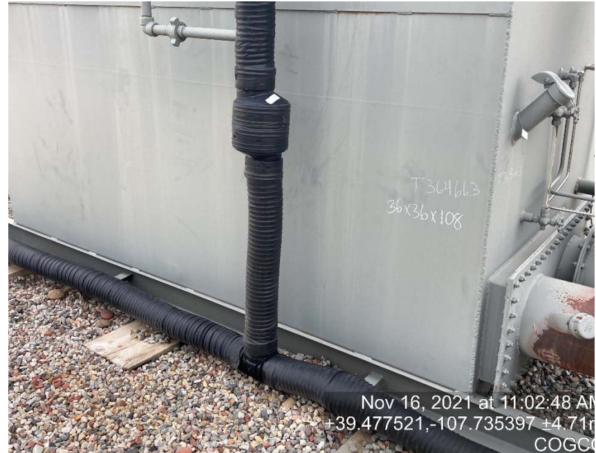
Glycol vessel lacking labeling
