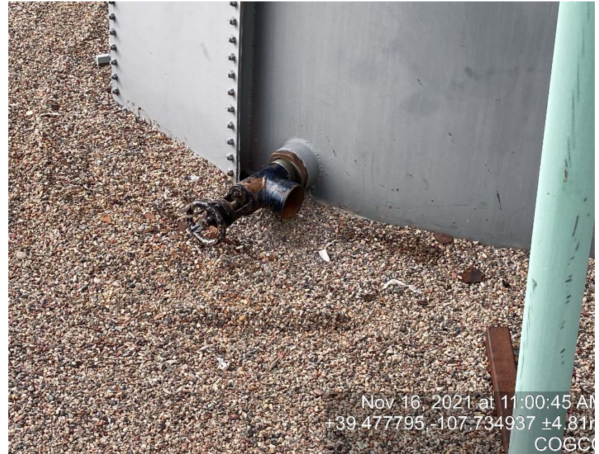
Load out lines lacking bull plugs/caps
