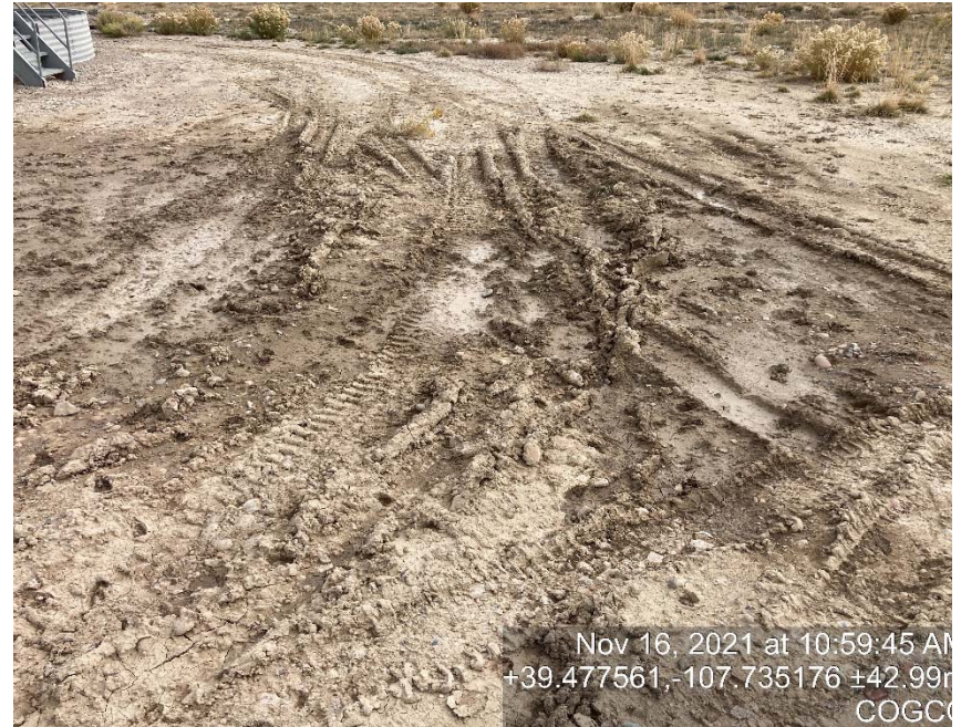
Lack of stabilization/compaction
