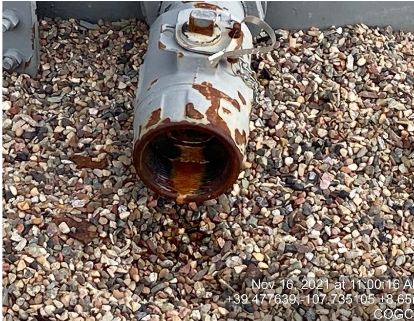
Load out lines lacking bull plugs/caps
