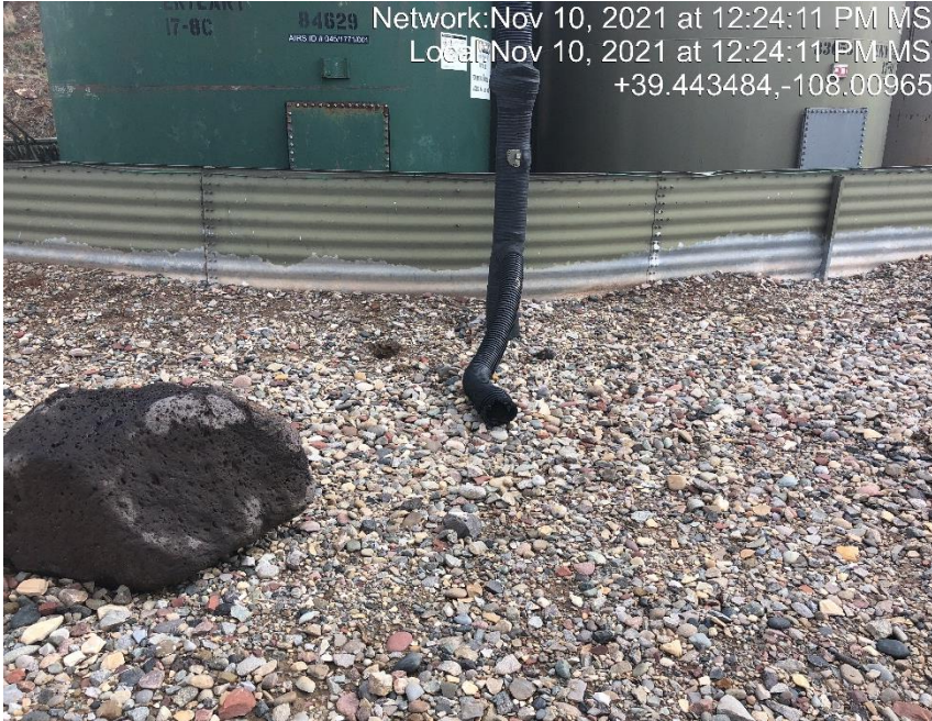
Photo #5183 Flowline heating insulation open ended and not capped.
