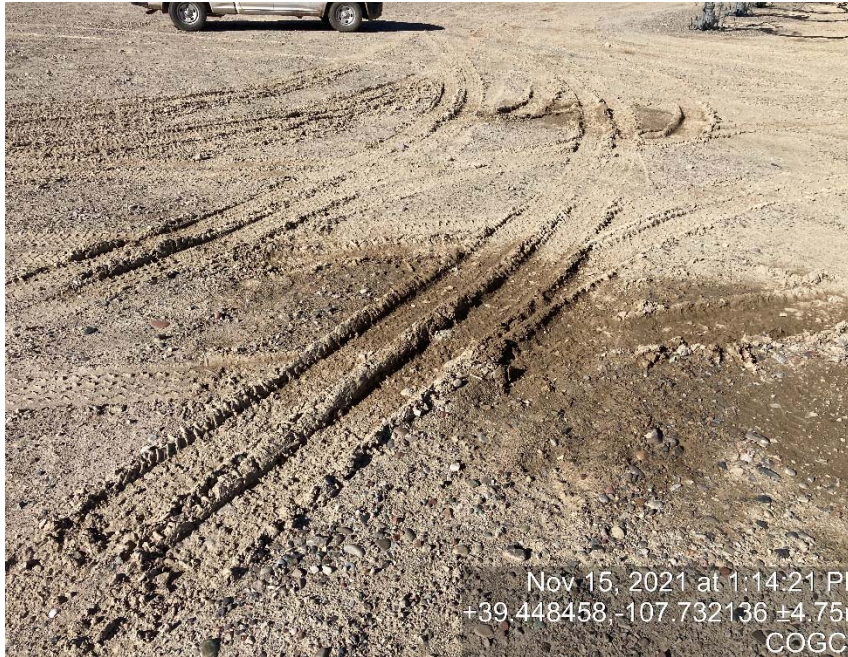
Lack of stabilization/compaction
