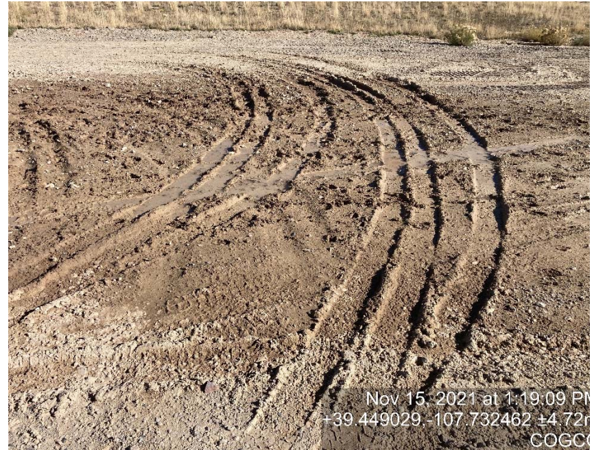
Lack of stabilization/compaction
