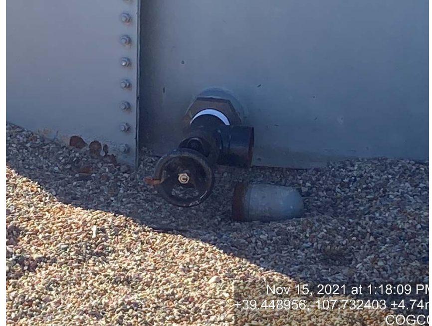
Load lines lacking bull plug
