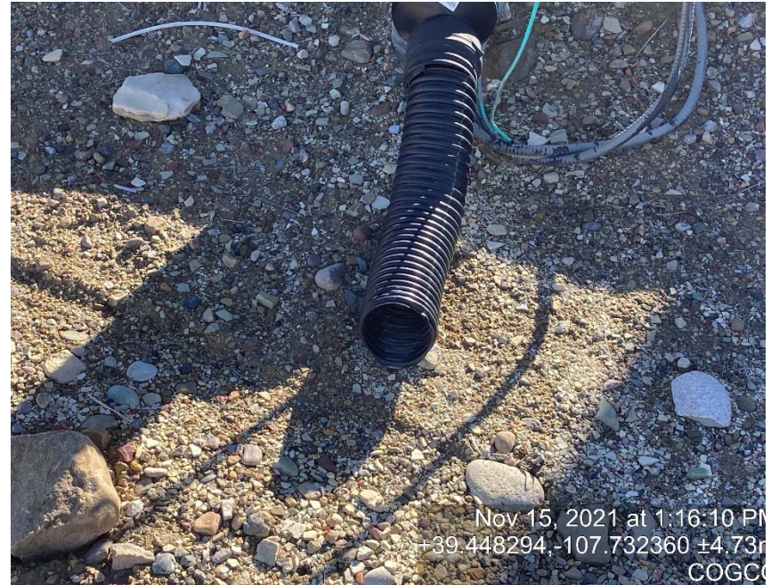
Open ended piping for thawing out dump lines on tanks with exhaust from trucks.
