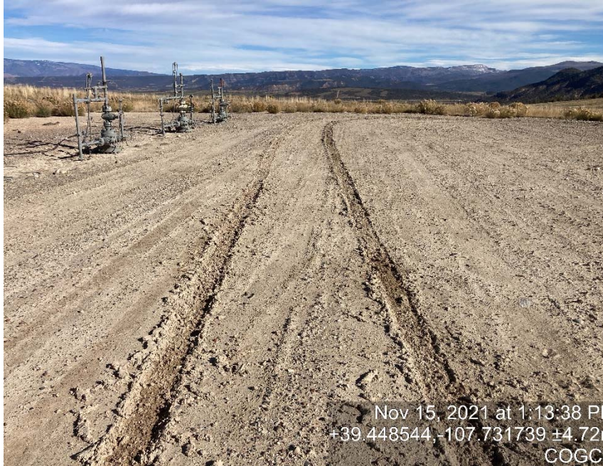
Lack of stabilization/compaction
