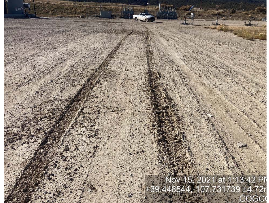
Lack of stabilization/compaction
