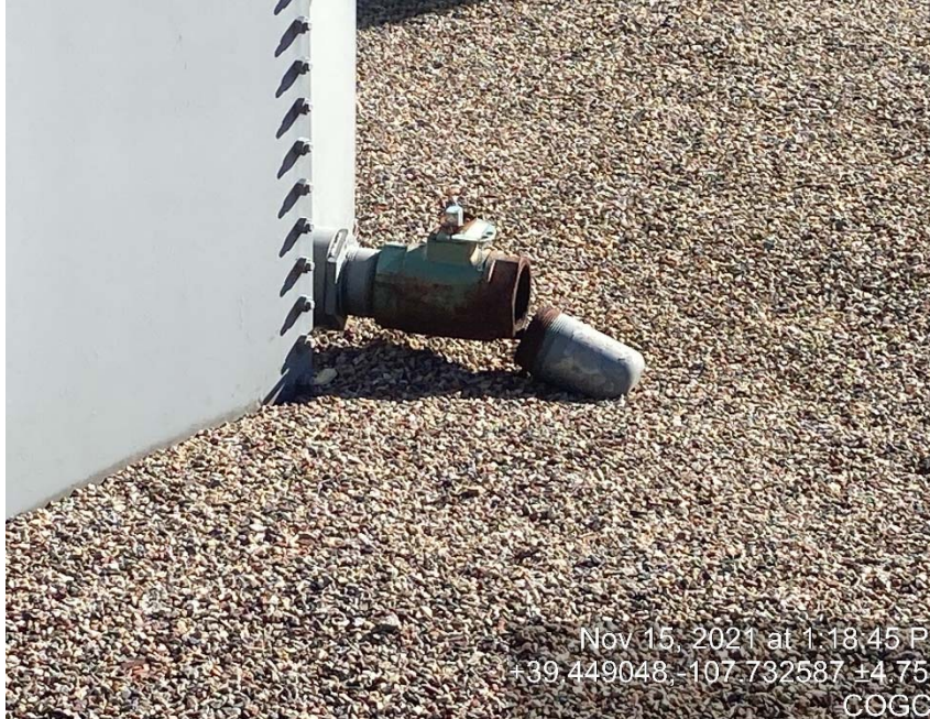
Load lines lacking bull plug
