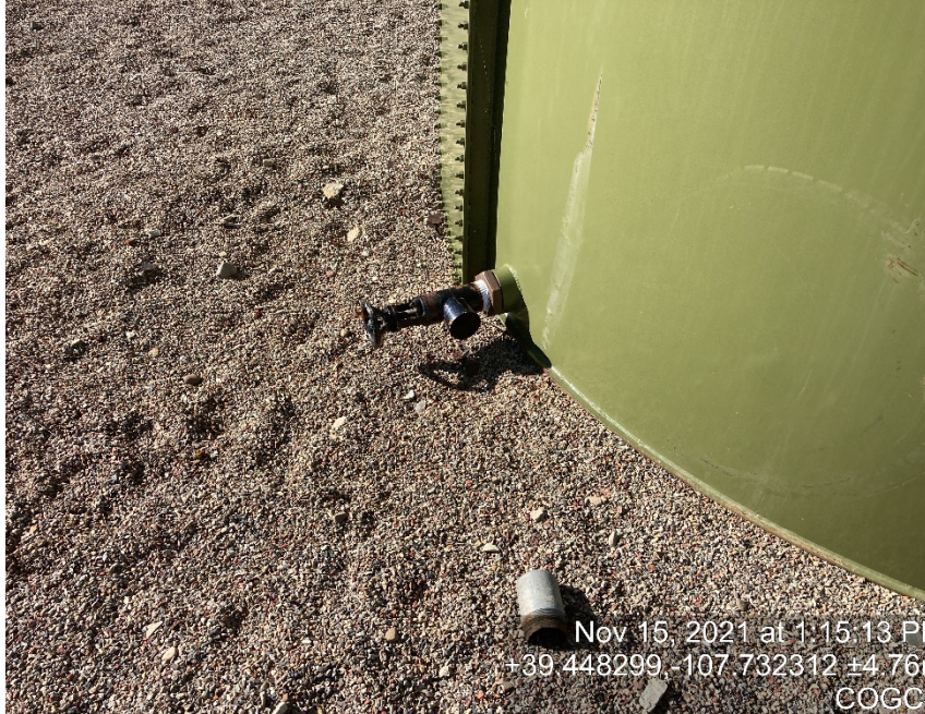
Load lines lacking bull plug
