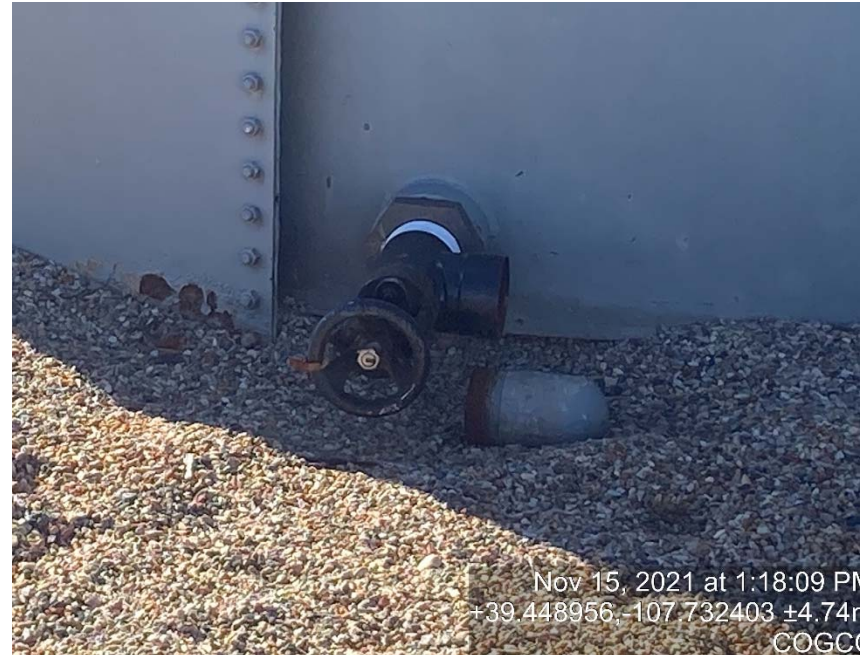
Load lines lacking bull plug
