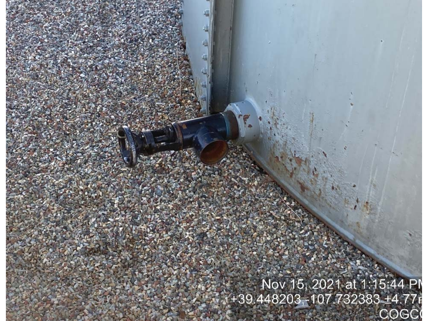
Load lines lacking bull plug
