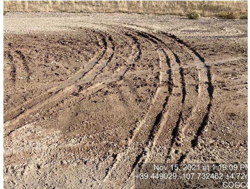
Lack of stabilization/compaction
