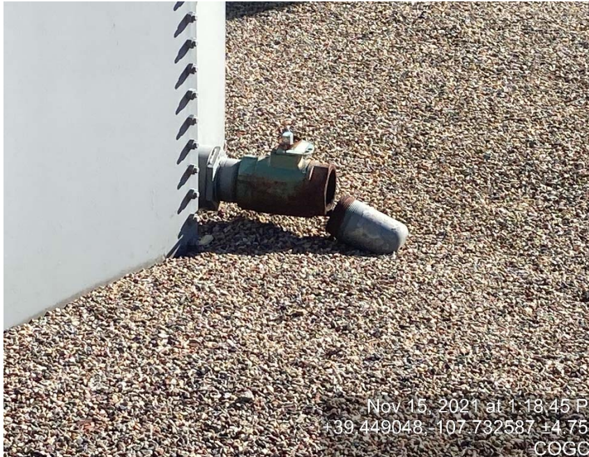
Load lines lacking bull plug
