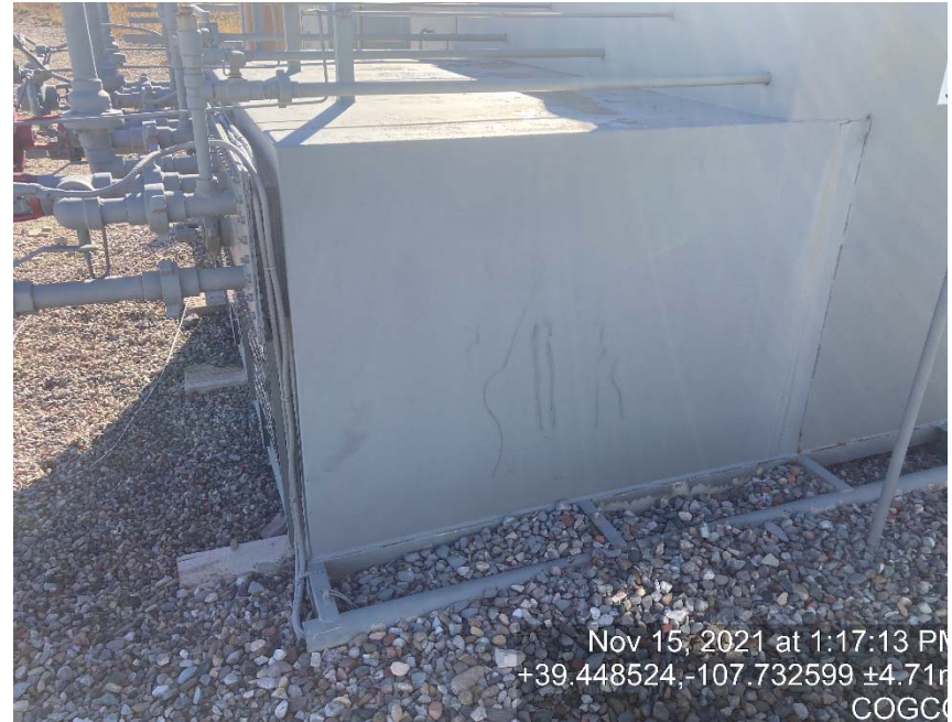
Glycol vessel lacking labeling
