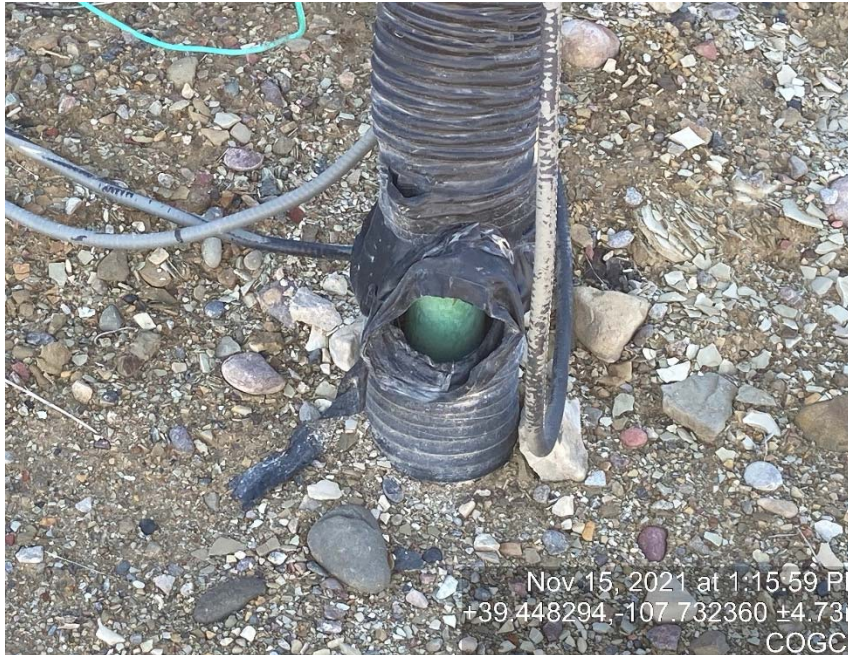
Open ended piping for thawing out dump lines on tanks with exhaust from trucks.
