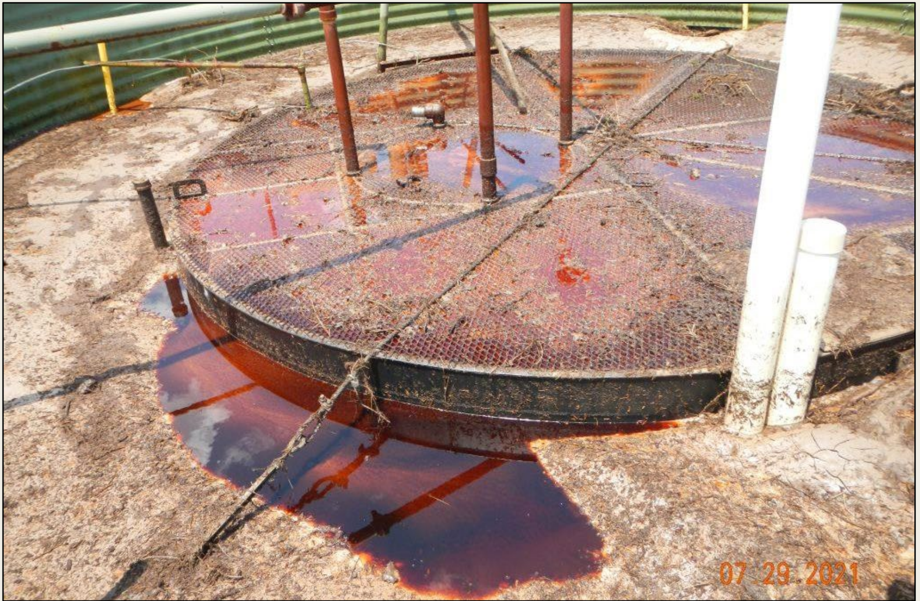
Photo 11. Another view of material released from overflowing tank.
