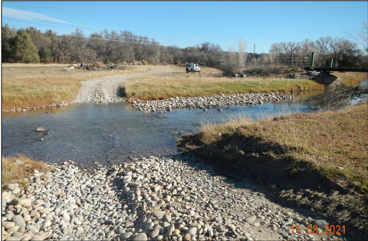
Photo 4. View of cobble placement within the low water crossing.
