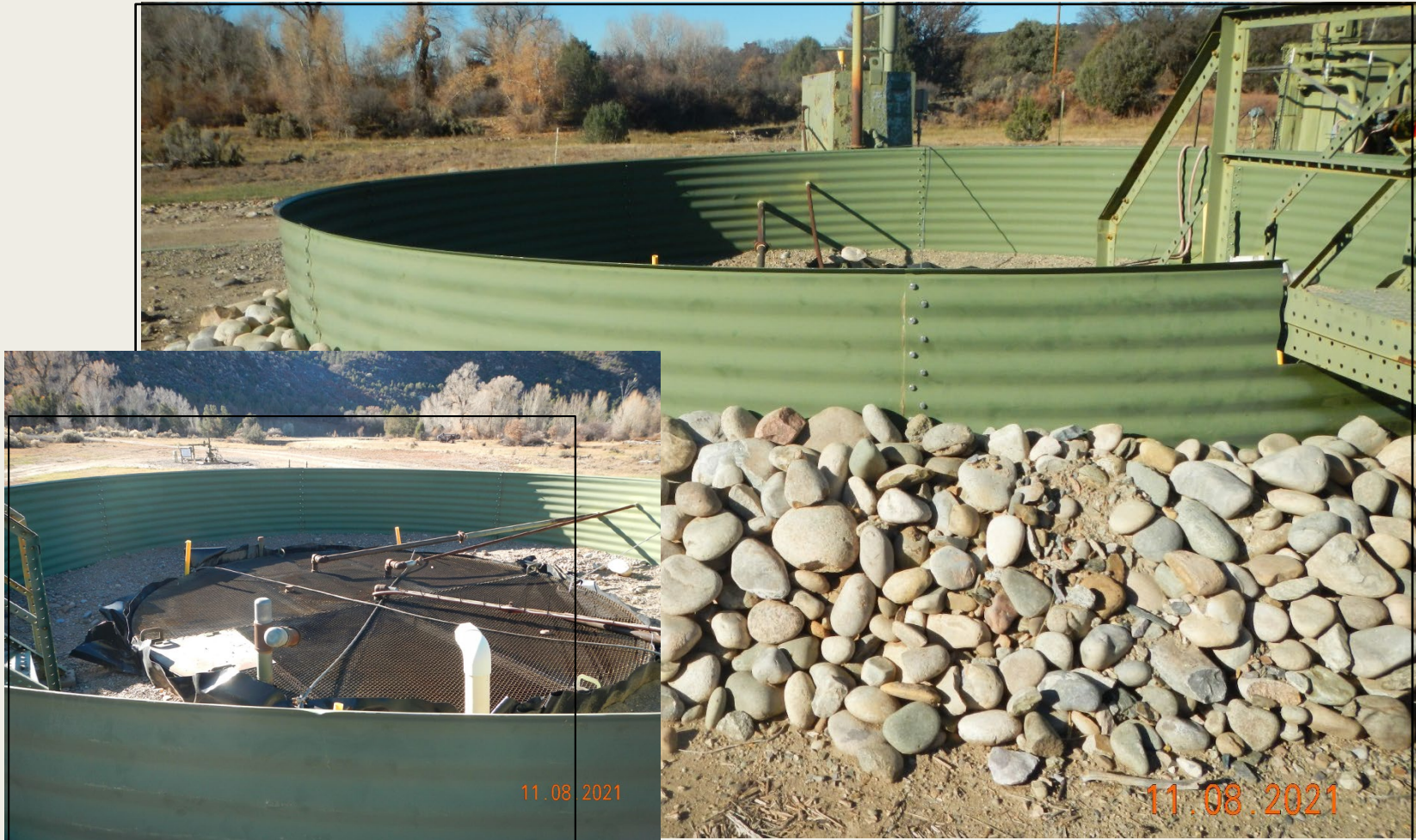
Photo 3. View of the partially buried vessel within the project area. Cobble placed around the base is not an adequate BMP. Vessel remains in place, approximately 6 inches above ground level (inset).
