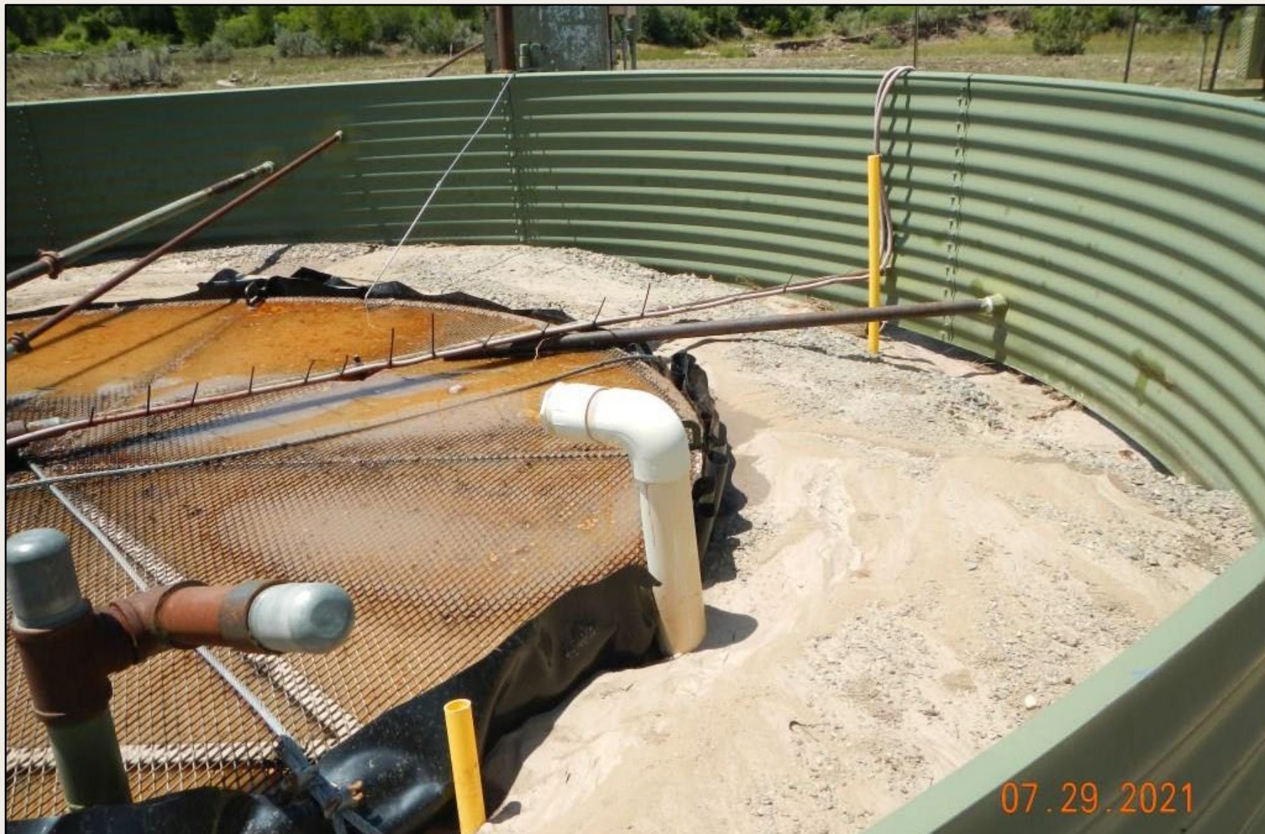
Photo 7. View of flow pattern from water flow due to compromised containment.
