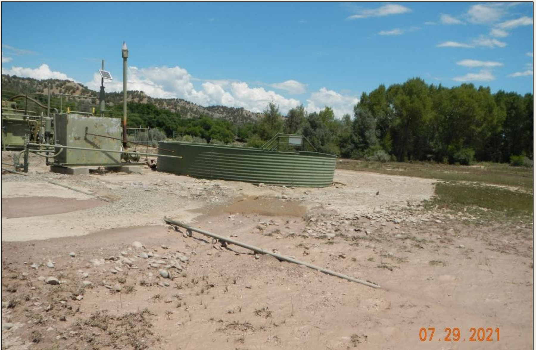
Photo 3. Another view of equipment facing upslope. Gravel is largely washed offsite.
