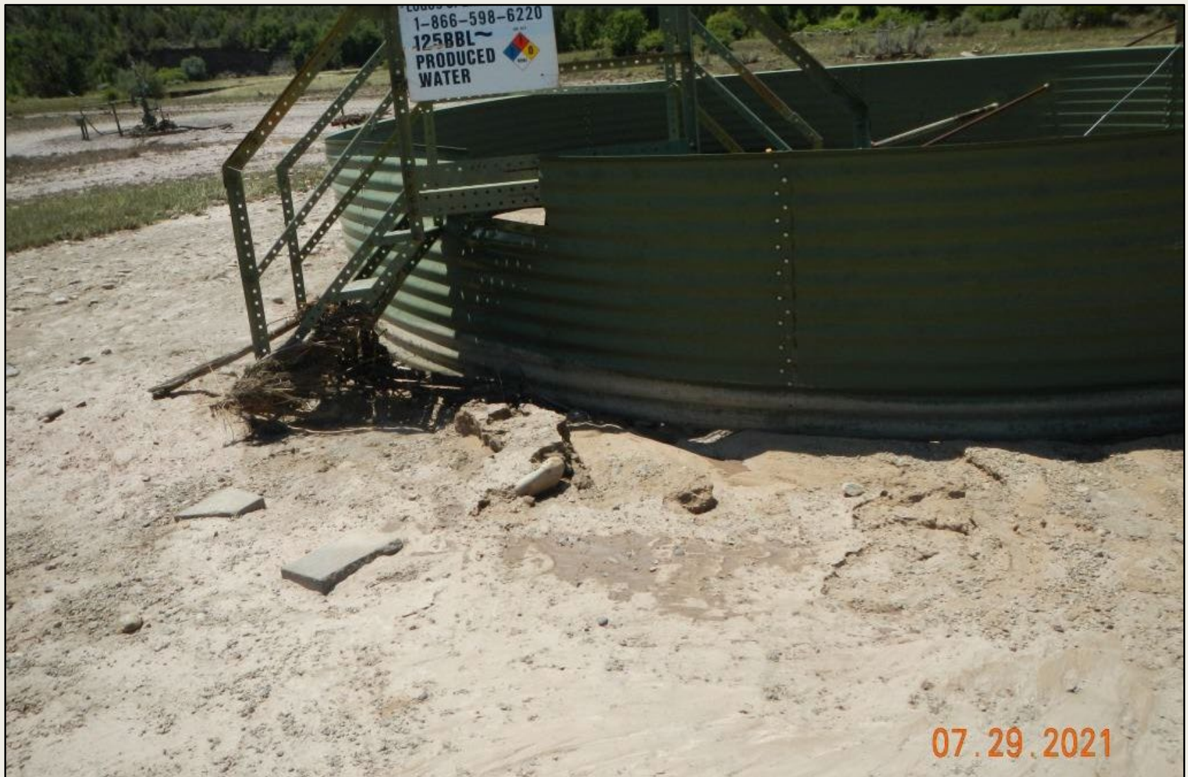
Photo 4. View of erosional scouring and flow pattern eroding beneath and around submerged vessel.
