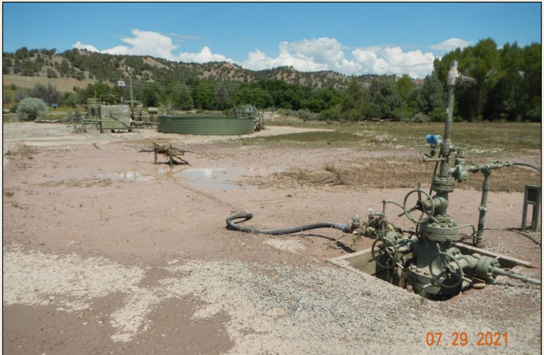
Photo 2. View of well and facilities. Stormwater has washed away material, exposing lines and deposited wood and plant debris on project facilities.
