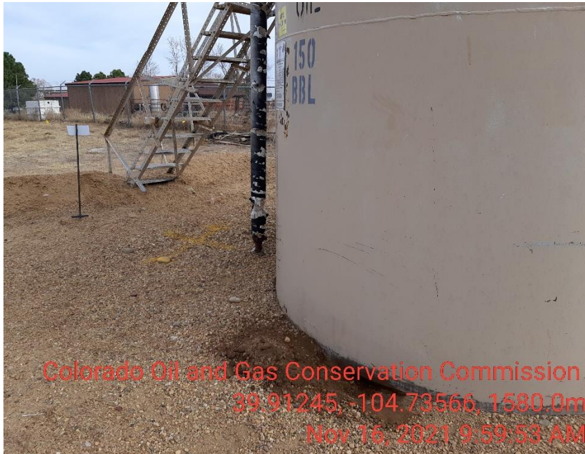
Photo 7 Stained soil around crude oil tank.
