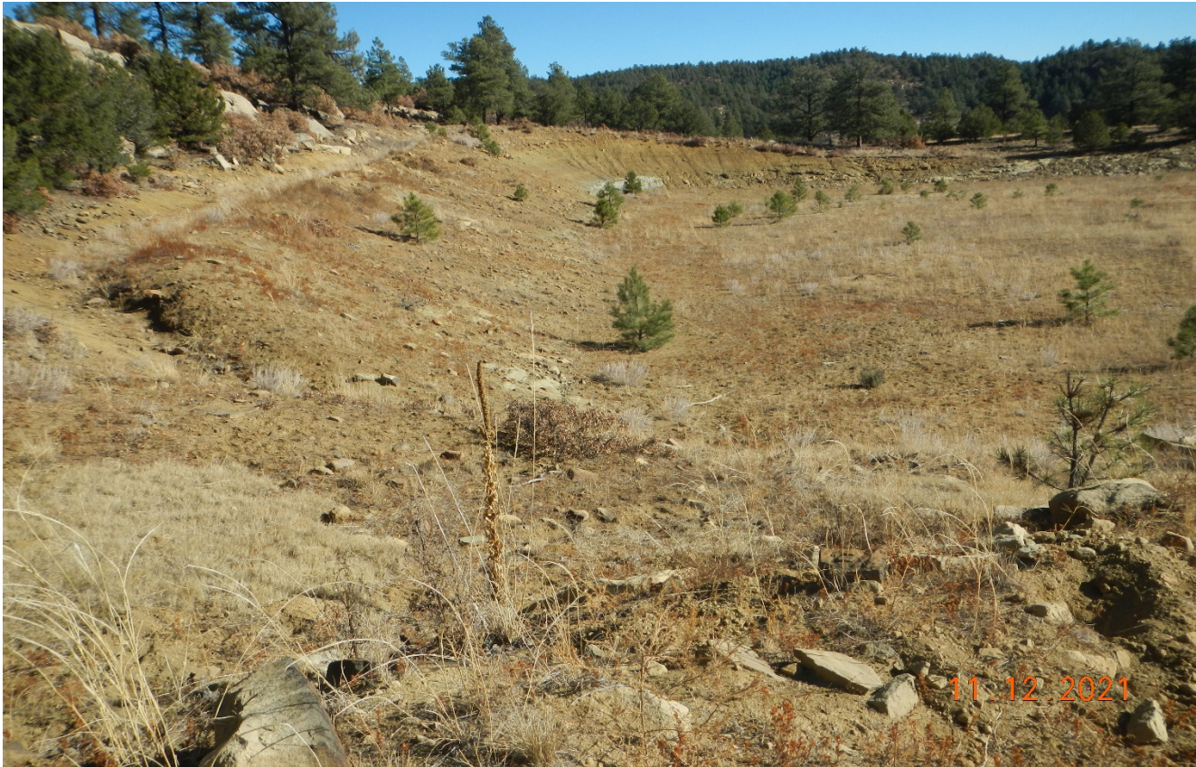
Photo 4. Facing northeast toward the location cut slope. The location has not been recontoured and reclaimed. The cut slope is not stabilized and there are signs of erosion.
