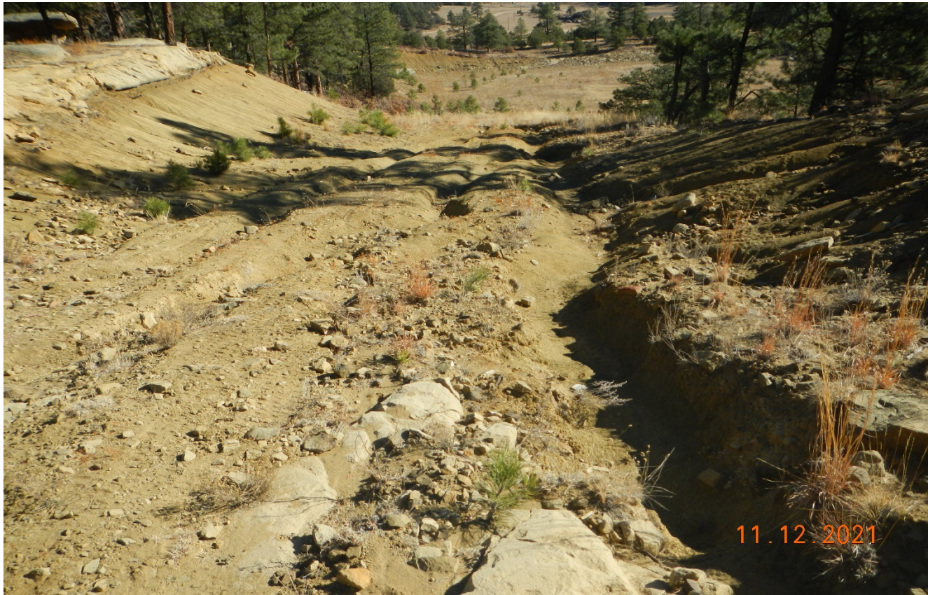
Photo 2. Facing east along the access road. There is erosion occurring down the road which is not stabilized. Previous correction action was not performed.
