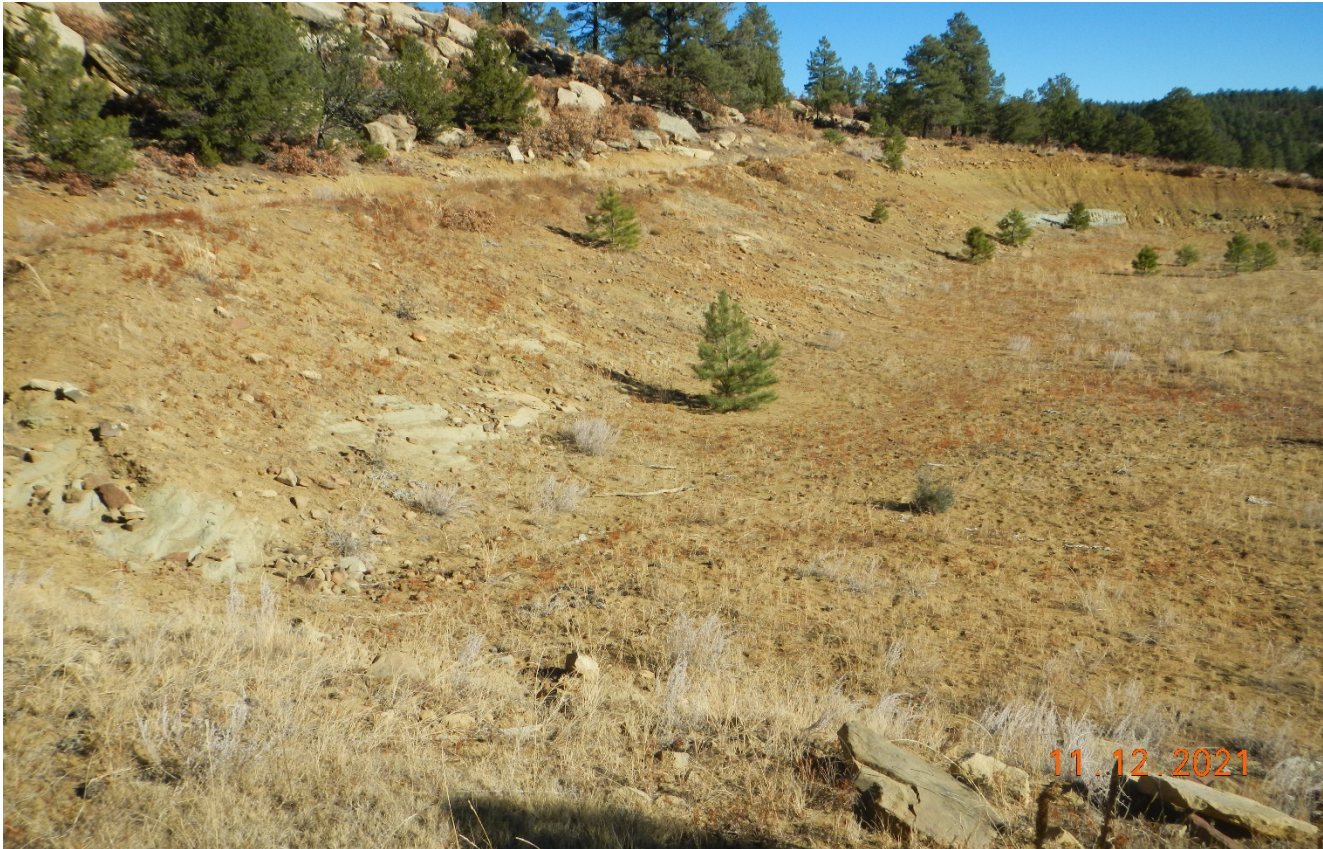
Photo 7. Facing toward the cut slope. The cut slope is not stabilized and there are signs of erosion.
