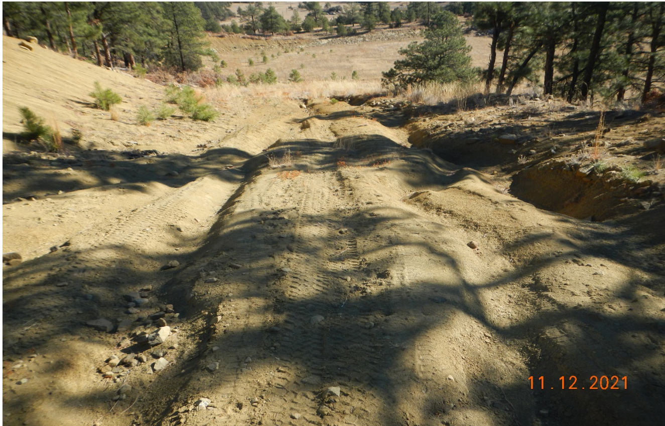
Photo 3. Facing east along the access road. There is erosion occurring down the road which is not stabilized. Previous correction action was not performed.
