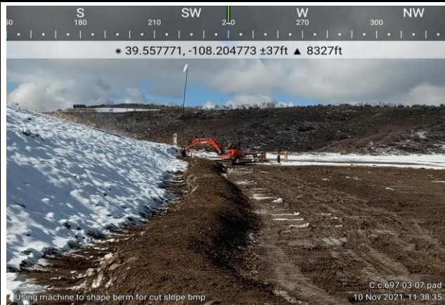
Installing Containment Berm below Cut Slope on Cascade Creek 697-03-07 Pad
