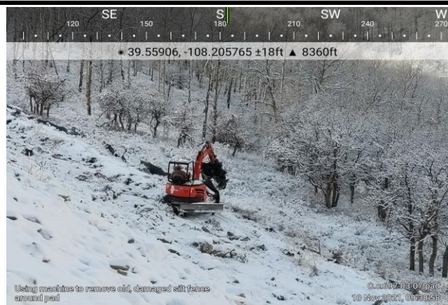
Replacing Damaged Silt Fence on Cascade Creek 697-03-07 Pad
