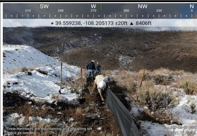
Replacing Damaged Silt Fence on Cascade Creek 697-03-07 Pad
