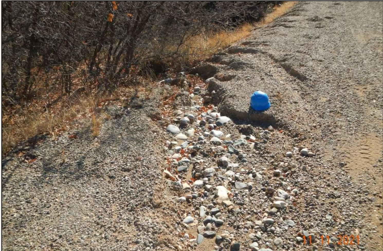
Photo 4. View of erosional channels and sediment transport occurring on the access road where and erosional channel flows down the well pad entrance and is eroding and discharging material down-slope from the project area. Erosion is approximately 1.5ft wide and up to 12 inches deep.
