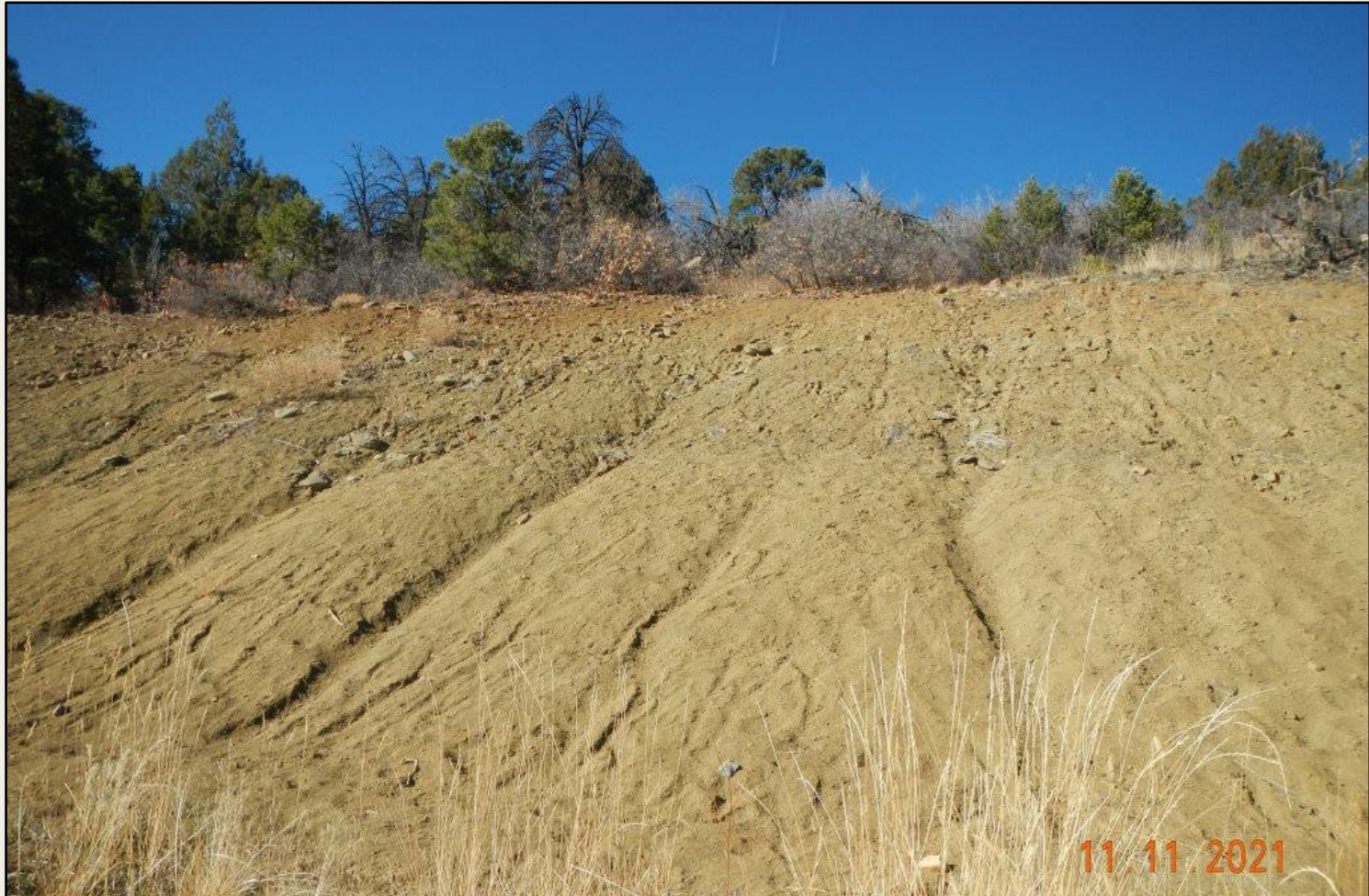
Photo 3. View of bare soils and erosional channels (approx. 10-12 inches wide and deep) on the well pad cut-slopes. .
