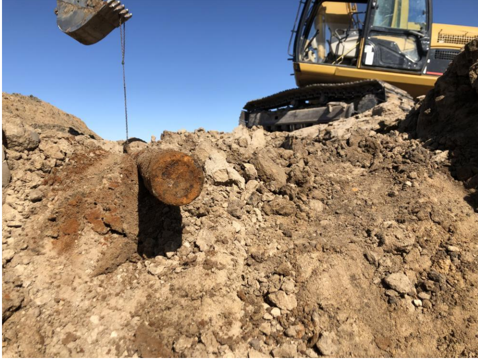
Capped gas equipment line following removal
