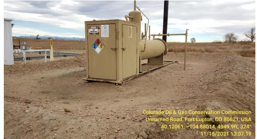
**Photo 5 flow line manifold**
