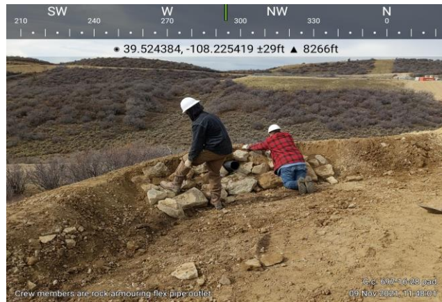
Installing Rock Armor Face on Flex Pipe Installation on Cascade Creek 697-16-28 Pad
