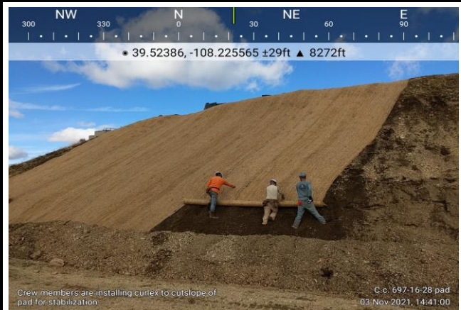
Installing Erosion Control Blankets on the CC 697-16-28 Pad
