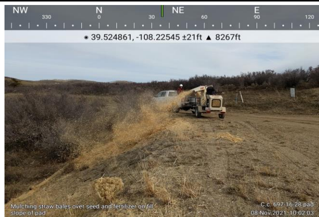
Applying Straw Mulch to Fill Slope on the Cascade Creek 697-16-28 Pad
