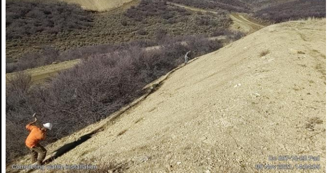
Installing Excelsior Wattle below Slopes on the CC 697-16-28 Pad
