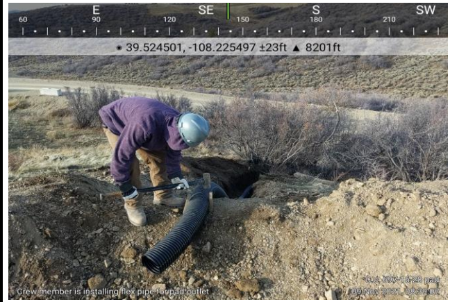
Installing Flex Pipe on Cascade Creek 697-16-28 Pad
