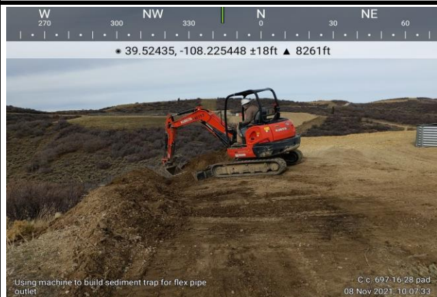
Installing Flex Pipe Outlet on the Cascade Creek 697-16-28 Pad
