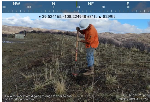
Hand Digging Test Holes on CC 697-16-28 Pad to Determine Topsoil Depth
