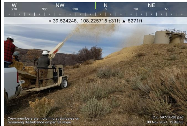
Applying Straw Mulch to Cascade Creek 697-16-28 Pad
