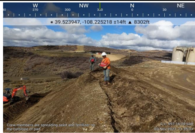
Broadcasting Seed and Fertilizer over the Erosion Control Blanket Installation
