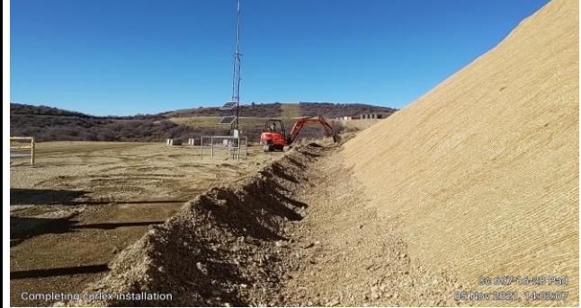
Installing Earthen Berm below Erosion Control Blanket Installations on CC 697-16-28 Pad
