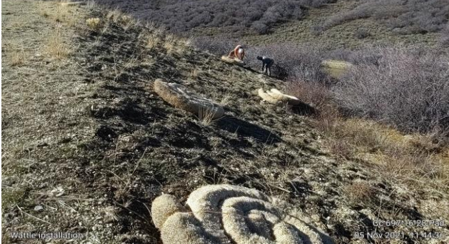
Installing Excelsior Wattle below Slopes on the CC 697-16-28 Pad
