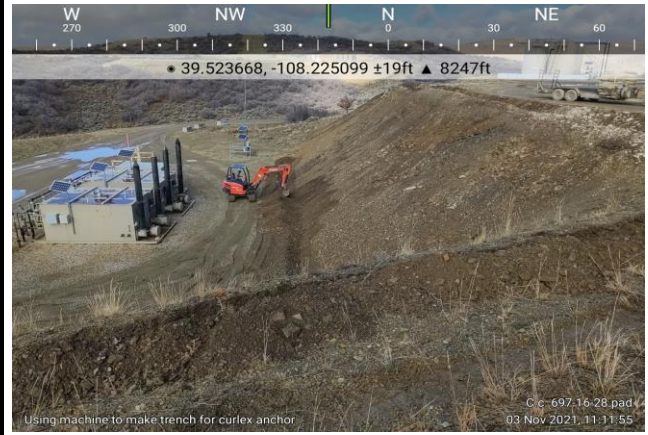
Installing Trench to Anchor Bottom of Erosion Control Blanket Installation
