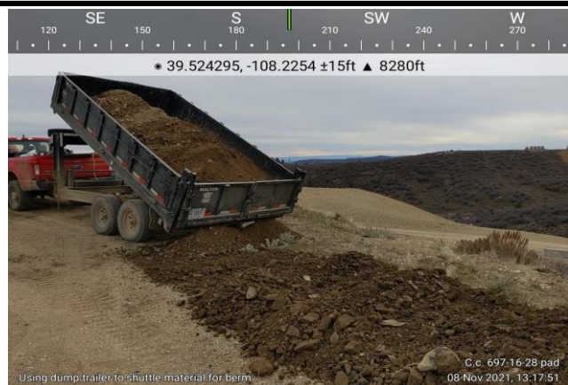
Delivering Material to Create a Flex Pipe Outlet on the Cascade Creek 697-16-28 Pad
