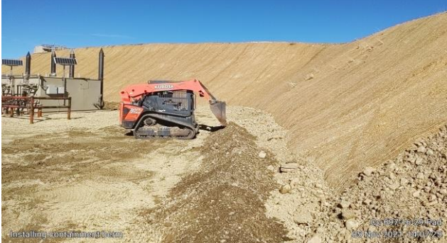
Installing Earthen Berm below Erosion Control Blanket Installations on CC 697-16-28 Pad
