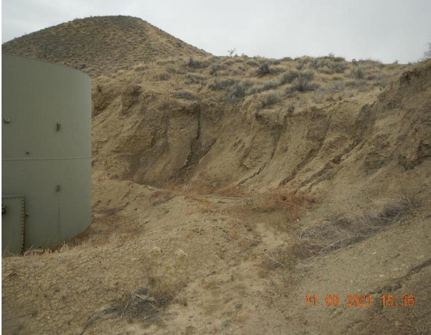
Unstable cutslope behind tank battery. Sediment built up to tank berm.
