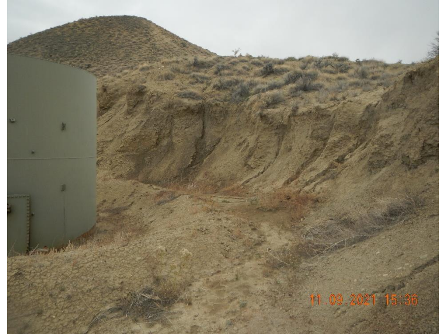
Unstable cutslope behind tank battery. Sediment built up to tank berm.
