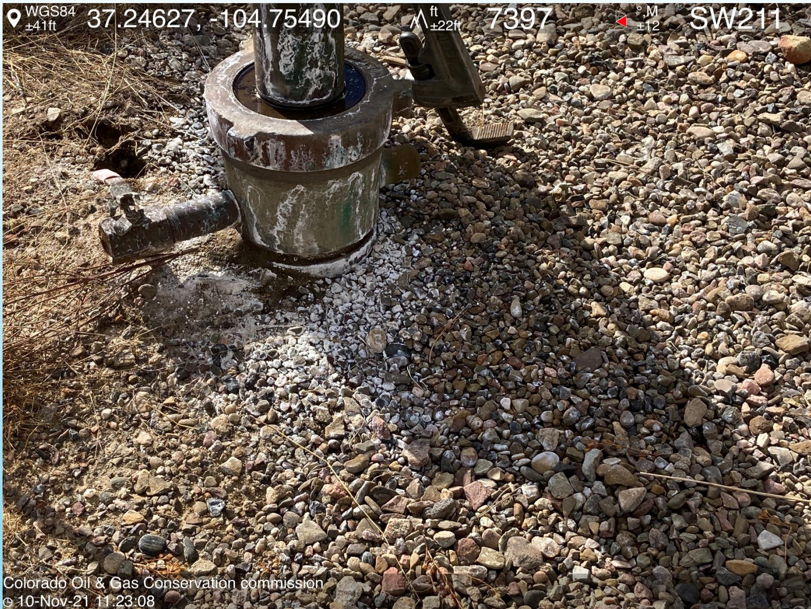
PHOTO 6: CLOSER IMAGE OF WHITE CHALKY BUILDUP AROUND TR WELLHEAD.
