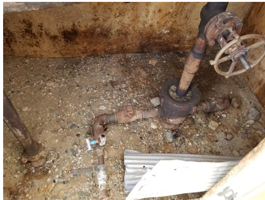
Photo 2. No bradenhead access apparent.
