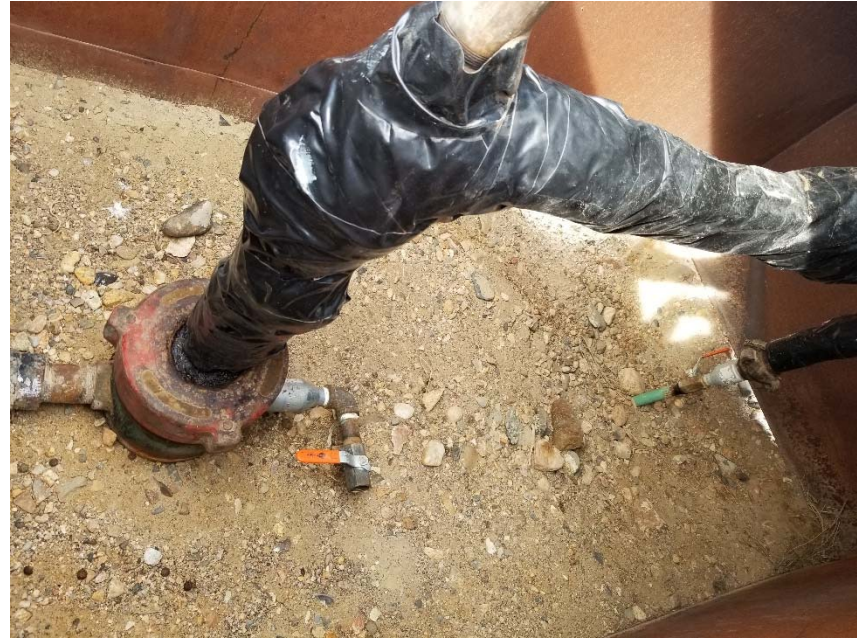
Photo 2. No bradenhead access apparent.
