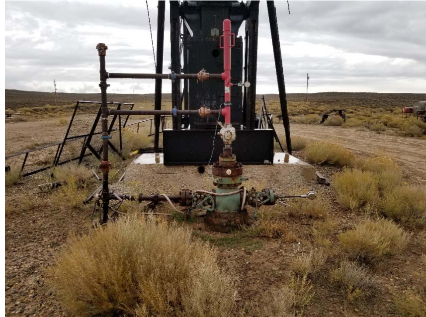
Photo 12. No wellhead sign. No bradenhead access apparent.
