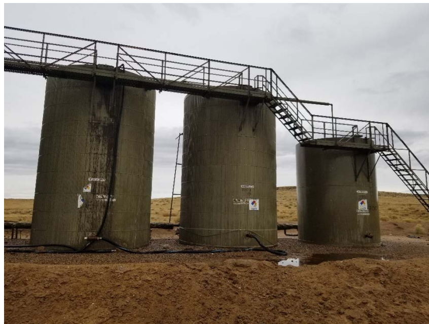
Photo 6. Missing and incomplete tank labels.
