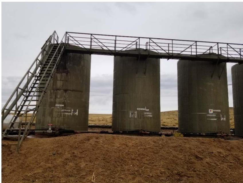
Photo 5. Missing and incomplete tank labels.
