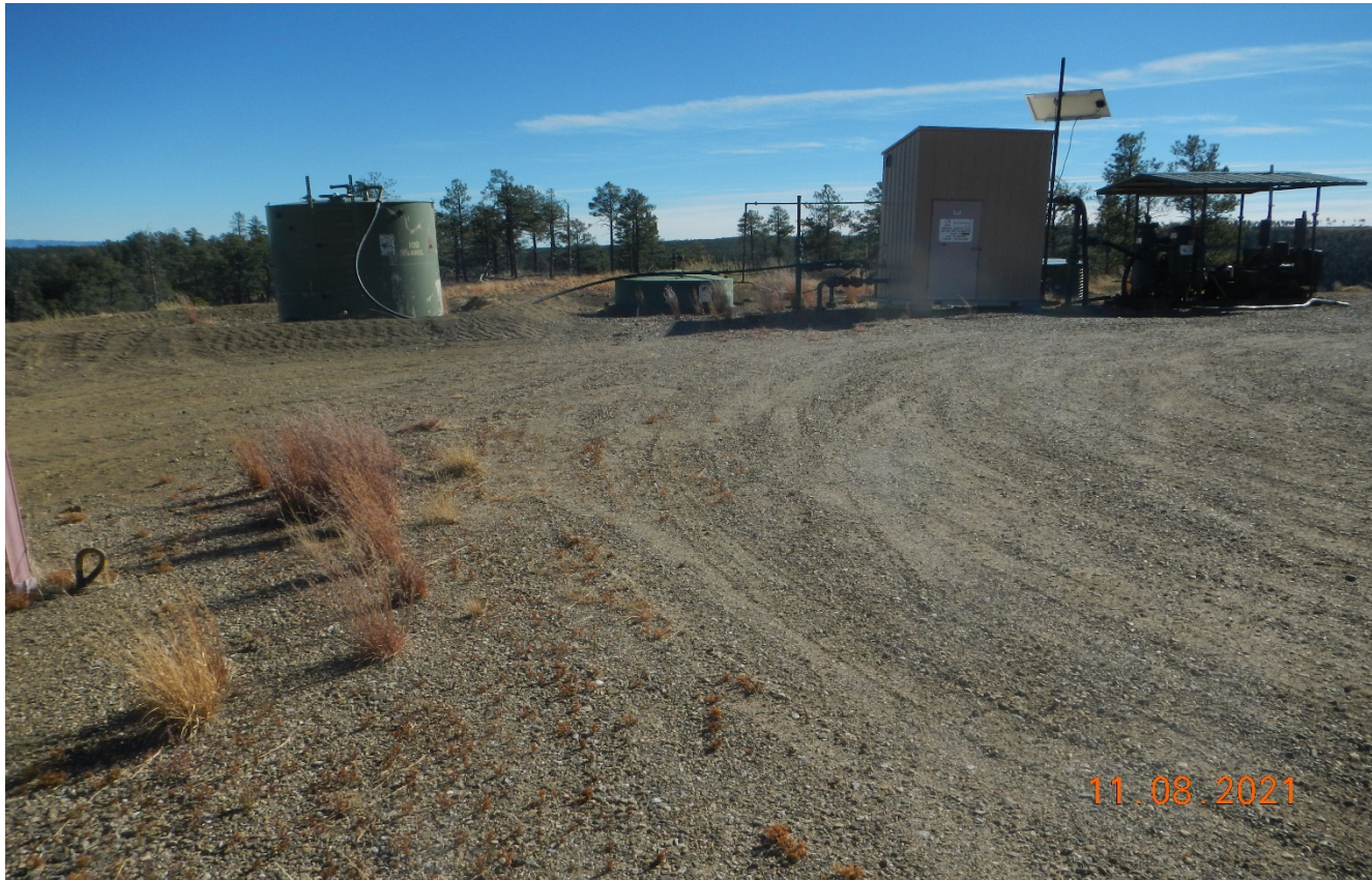
Photo 2. The berm around the tank has been repaired.
