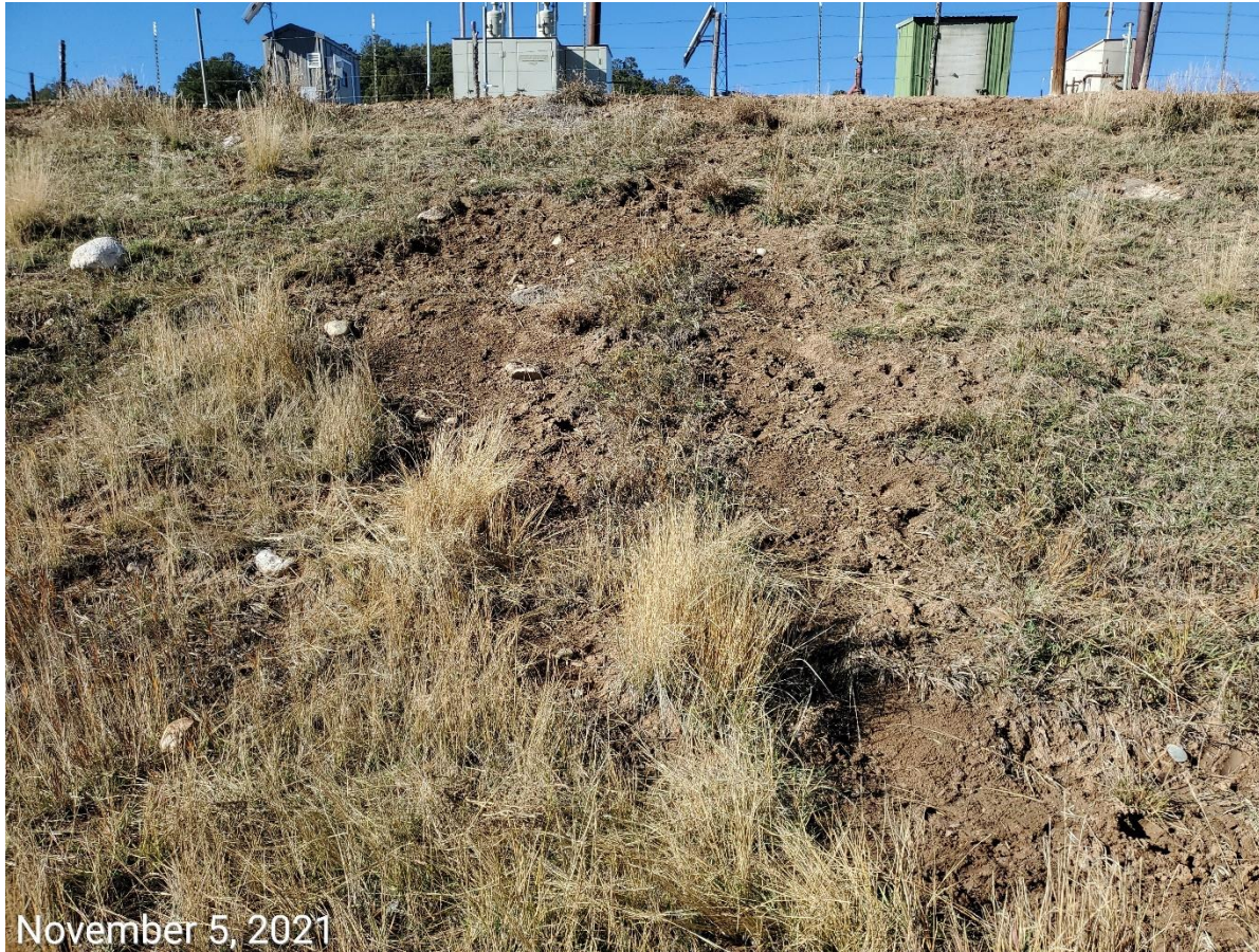
Photo 1: Photo shows erosion degradation at the fill slope; photo shows stormwater and erosion control measures remain missing or insufficient.
