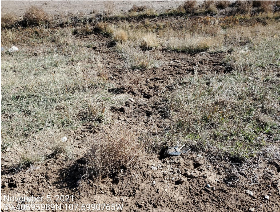
Photo 2: Photo shows erosion degradation at the fill slope; photo shows stormwater and erosion control measures remain missing or insufficient.
