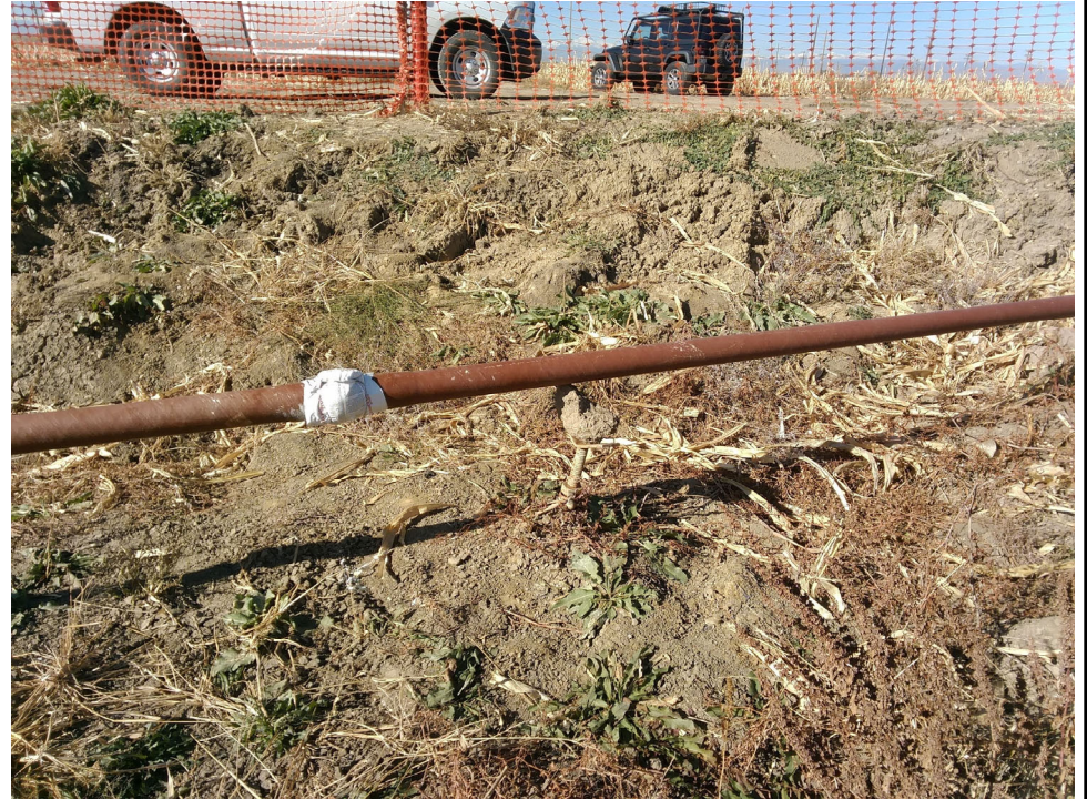
View of new fiberglass replacement section supported by angular rock on top of screw-type pipe support. In lieu of embedment into backfill.
