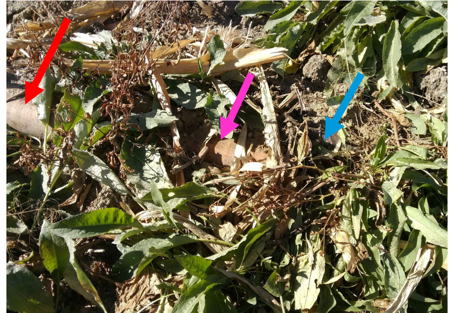
View of two improperly abandoned lines. Pink and blue arrows appear to be two split ends of the same line as both are visibly open-ended.
