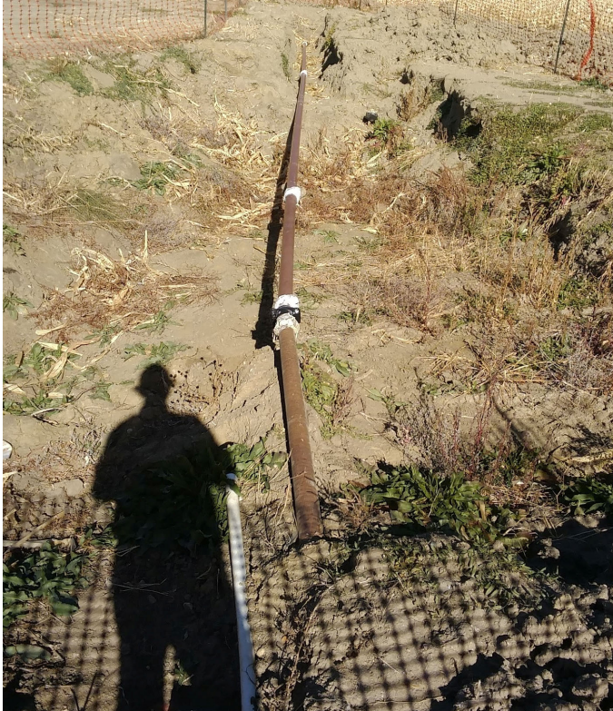
View of slight bowing at the southern tie-in with stub end. There is no embedment into soil.
