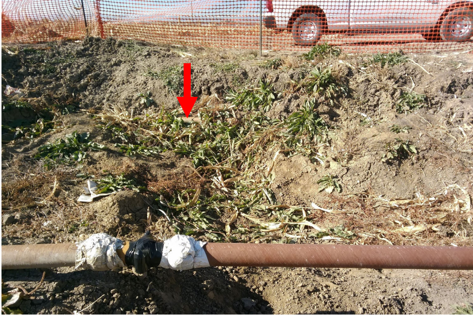
View of west edge of larger excavation area containing improperly abandoned lines. Red arrow is partial exposure of one of the two lines in question.
