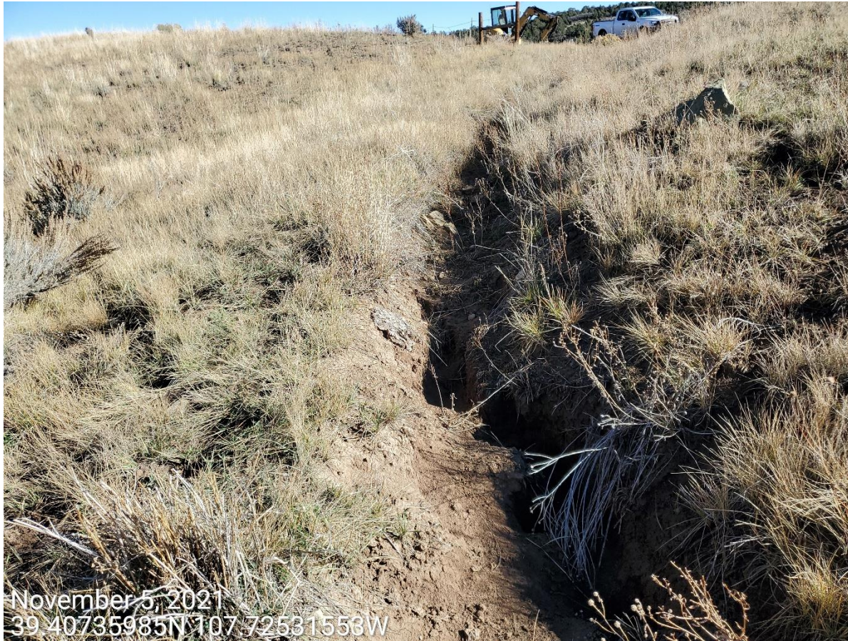
Photo 5: Photo taken from the stormwater diversion ditch southwest from the Location and the sediment trap; erosion degradation and incising due to stormwater runoff evident within ditch; control measures have not been constructed per good engineering practices or maintained in proper functioning condition
