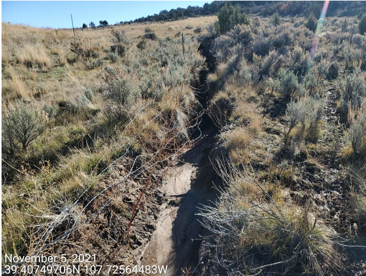
Photo 10: Photo shows gully erosion due to inadequate stormwater and erosion control measures, and improper stormwater discharge from the Location.
