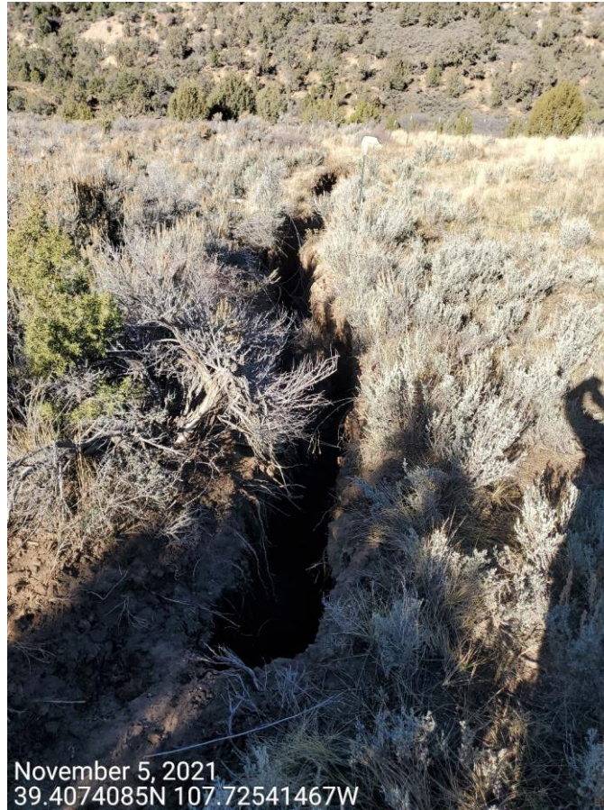
Photo 8: Continued from photo 7. Photo shows gully erosion due to inadequate stormwater and erosion control measures, and improper stormwater discharge from the Location.
