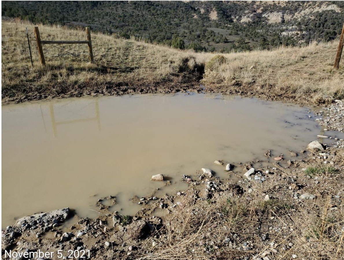
Photo 4: Photo taken from the sediment trap on the southwest end of the Location; stormwater discharge from the trap continues into a stormwater diversion ditch that travels southwest of the Location. Photo shows control measure has not been constructed with an appropriate outlet in accordance with good engineering practices.
