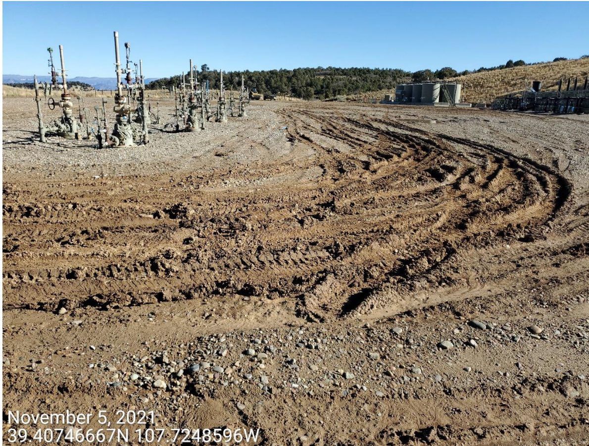
Photo 1: Photos 1-3 taken from the production areas of the Location. Photos provide examples showing that control measures to stabilize, mitigate tracking and offsite sediment transport at the production areas of the Location are missing or insufficient.
