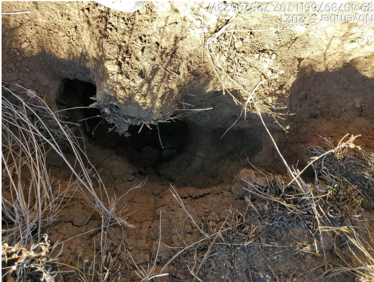
Photo 6: Continued from photo 5. Photo shows erosion degradation within the ditch.
