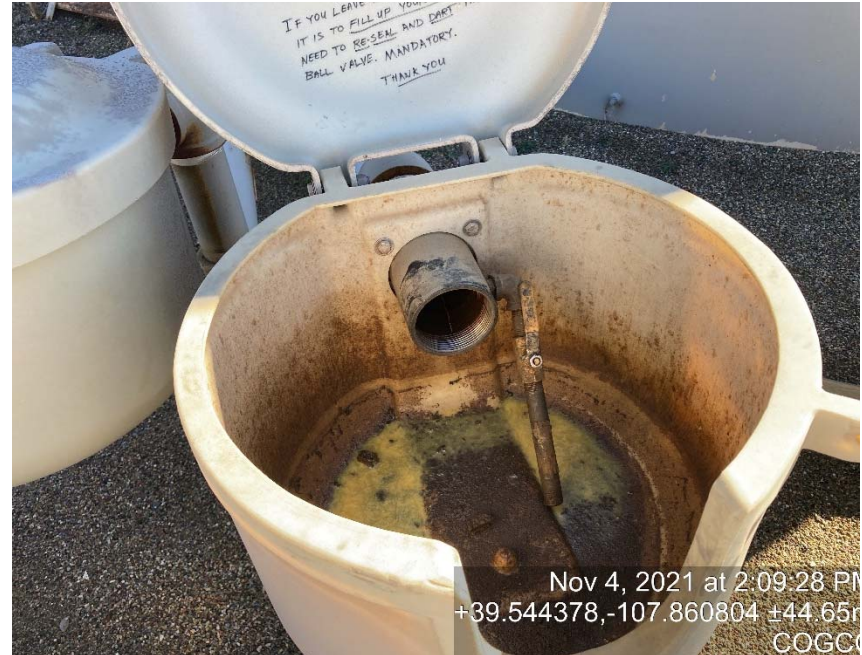
Load lines missing bull plugs/caps
