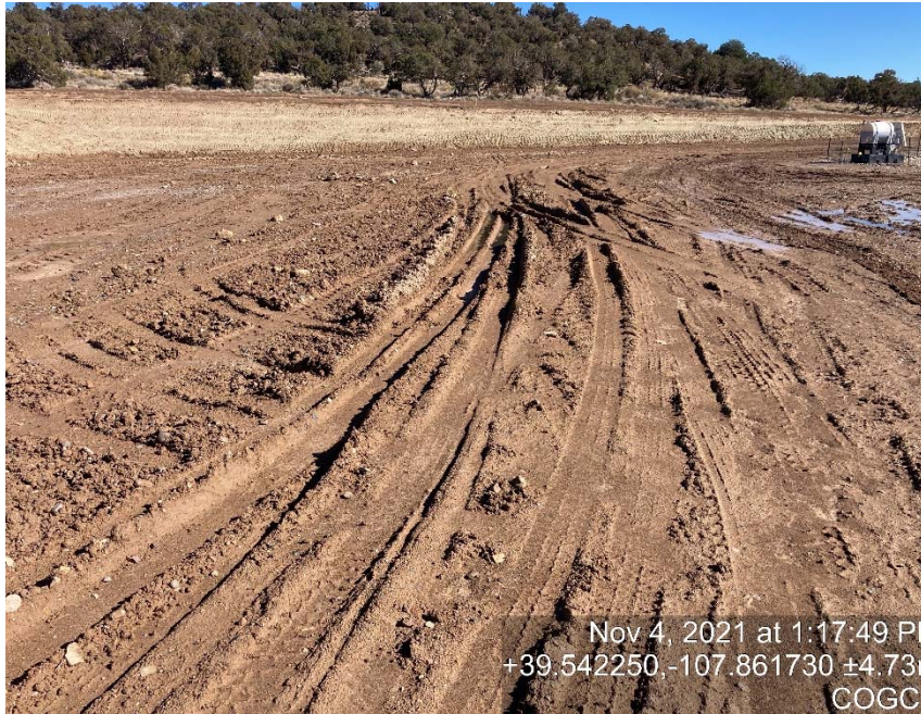
Lack of stabilization/compaction
