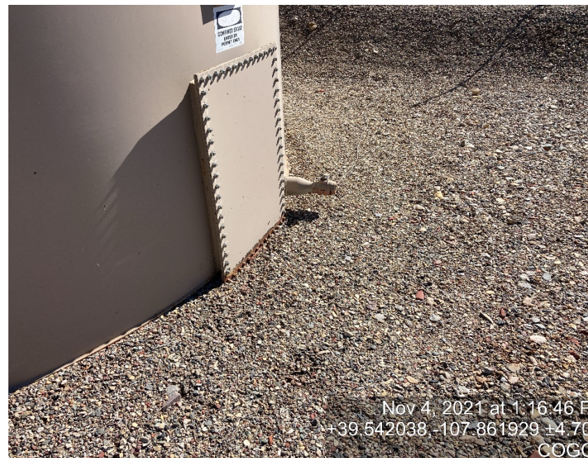
Load line missing bull plug/cap
