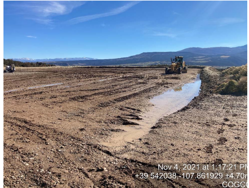
Lack of stabilization/compaction
