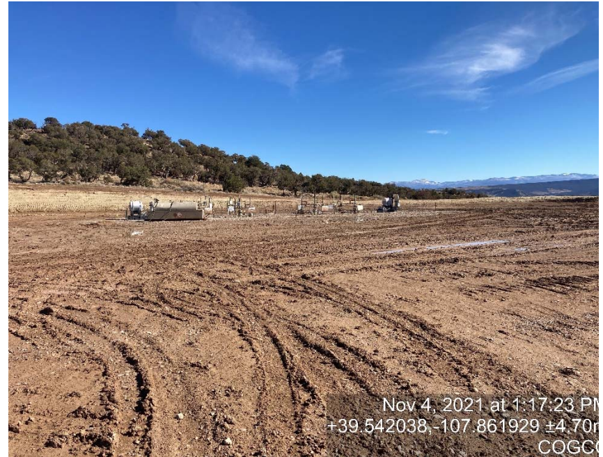
Lack of stabilization/compaction
