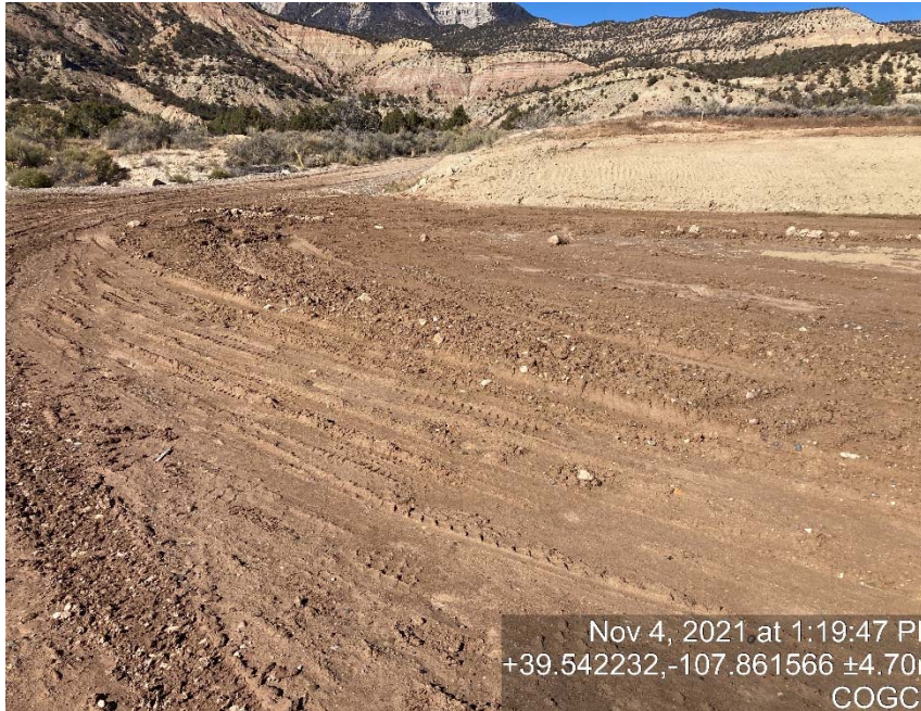
Lack of stabilization/compaction
