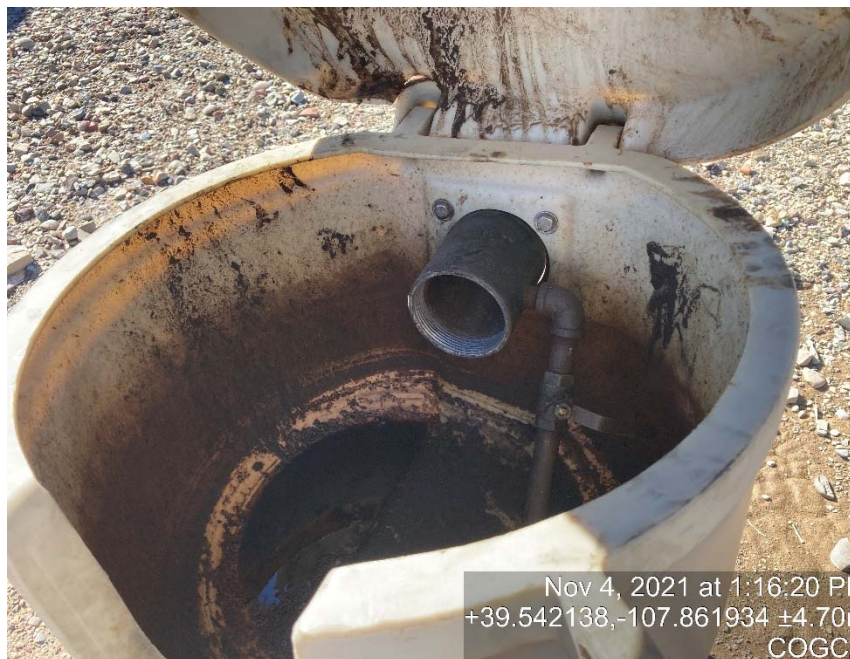
Load line missing bull plug/cap
