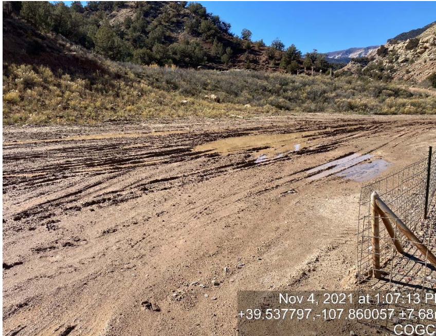
Lack of stabilization/compaction
