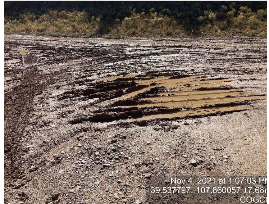
Lack of stabilization/compaction
