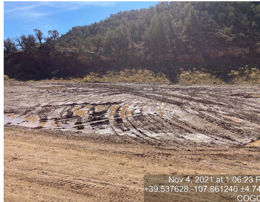
Lack of stabilization/compaction
