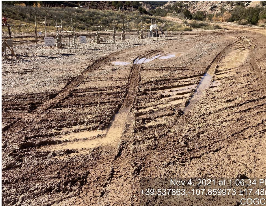
Lack of stabilization/compaction
