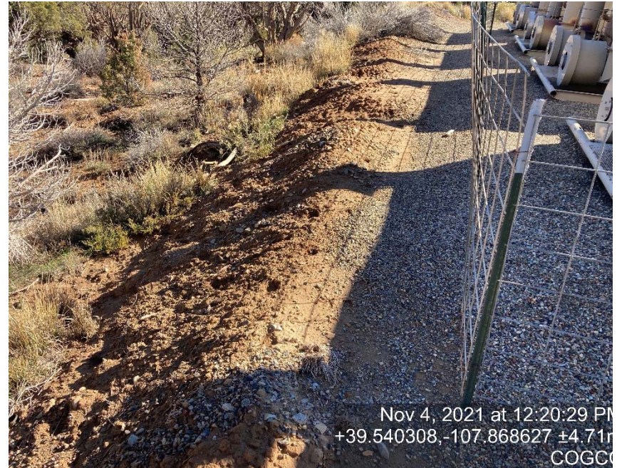
Erosion/sediment migration behind separators
