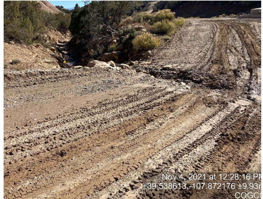
Access road drainage crossing needs maintained
