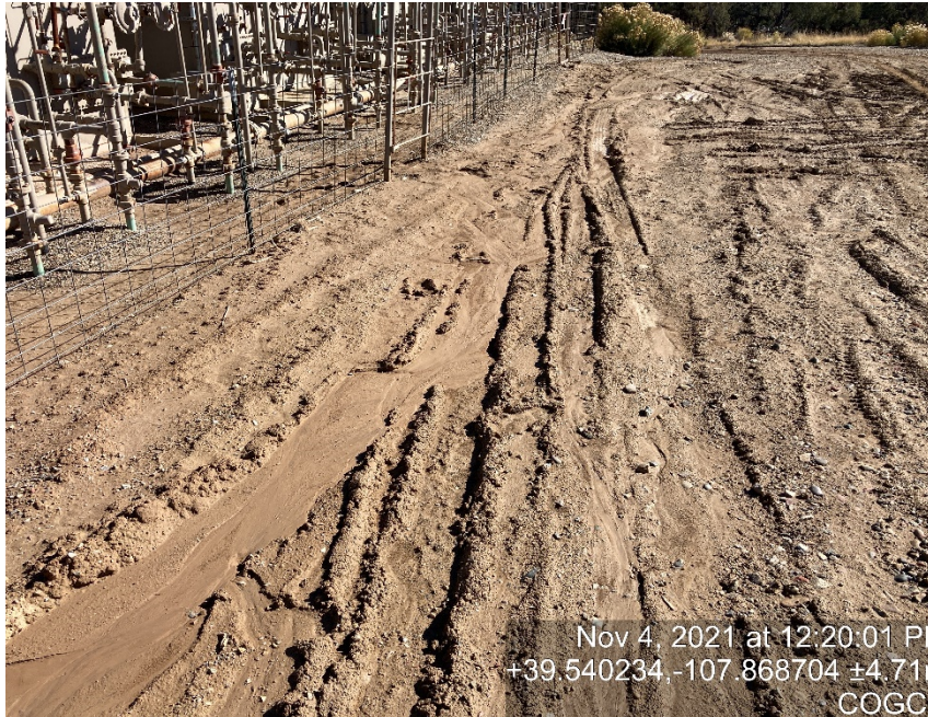
Lack of stabilization/compaction
