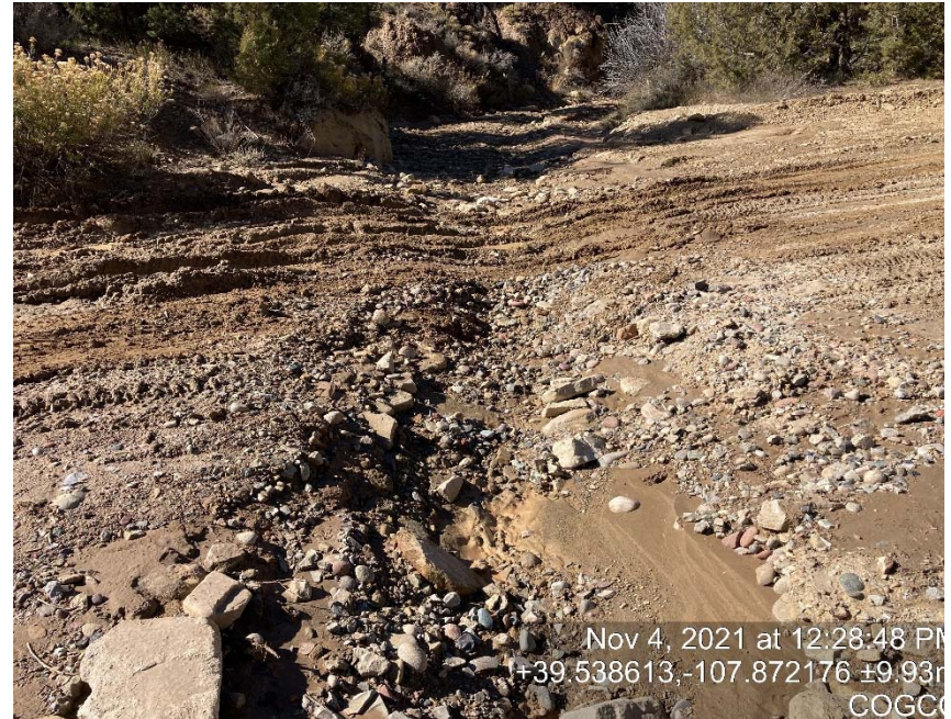
Access road drainage crossing needs maintained
