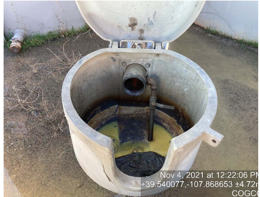
Load line missing bull plug/cap
