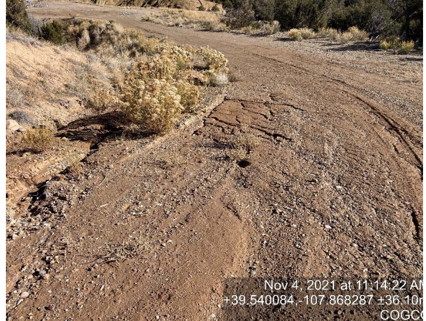
Erosion on access to wells
