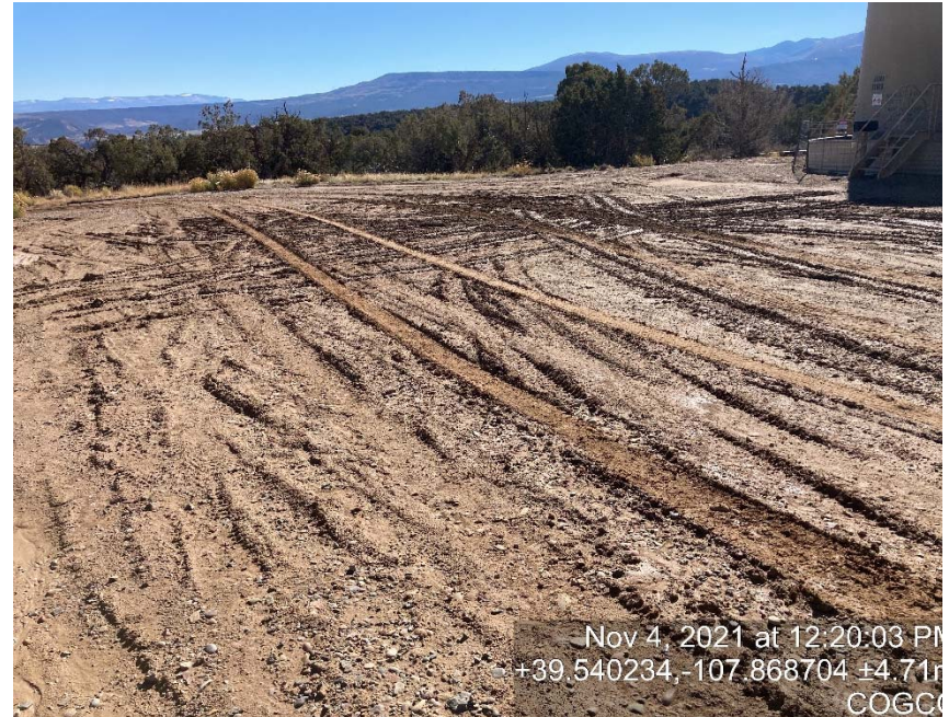
Lack of stabilization/compaction
