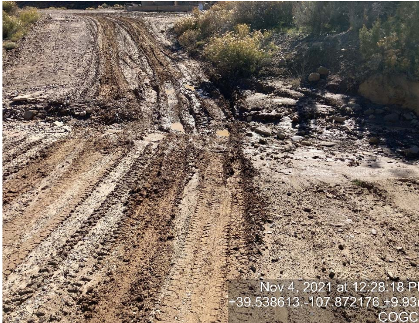
Access road drainage crossing needs maintained
