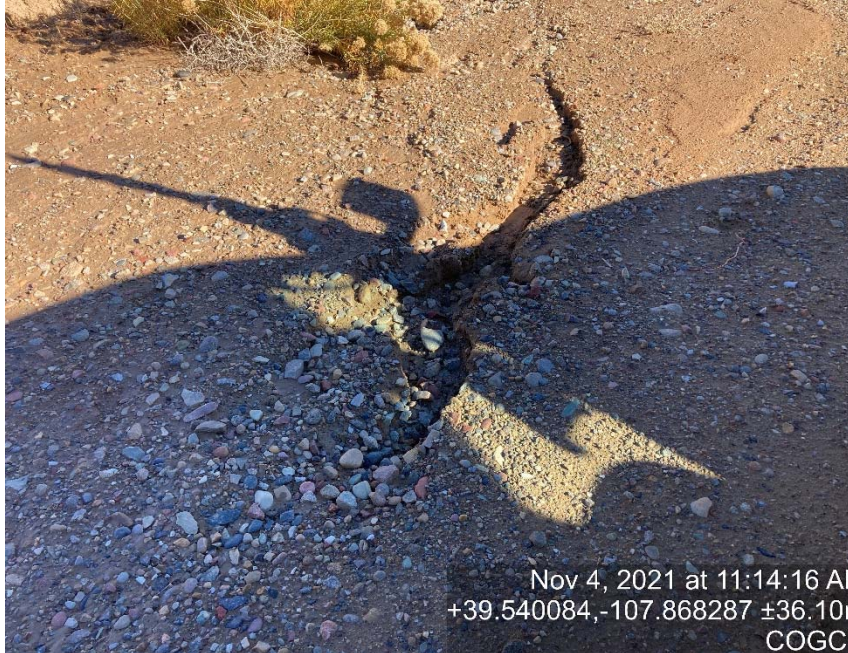
Erosion on access to wells
