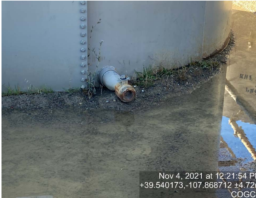
Load line missing bull plug/cap
