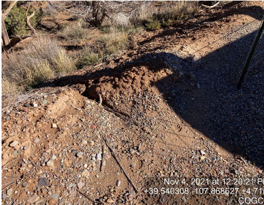
Erosion/sediment migration behind separators
