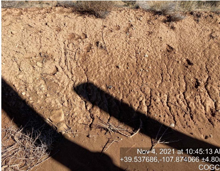
Lack of stabilization/erosion
