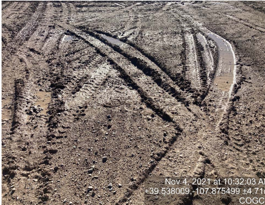
Lack of stabilization/compaction
