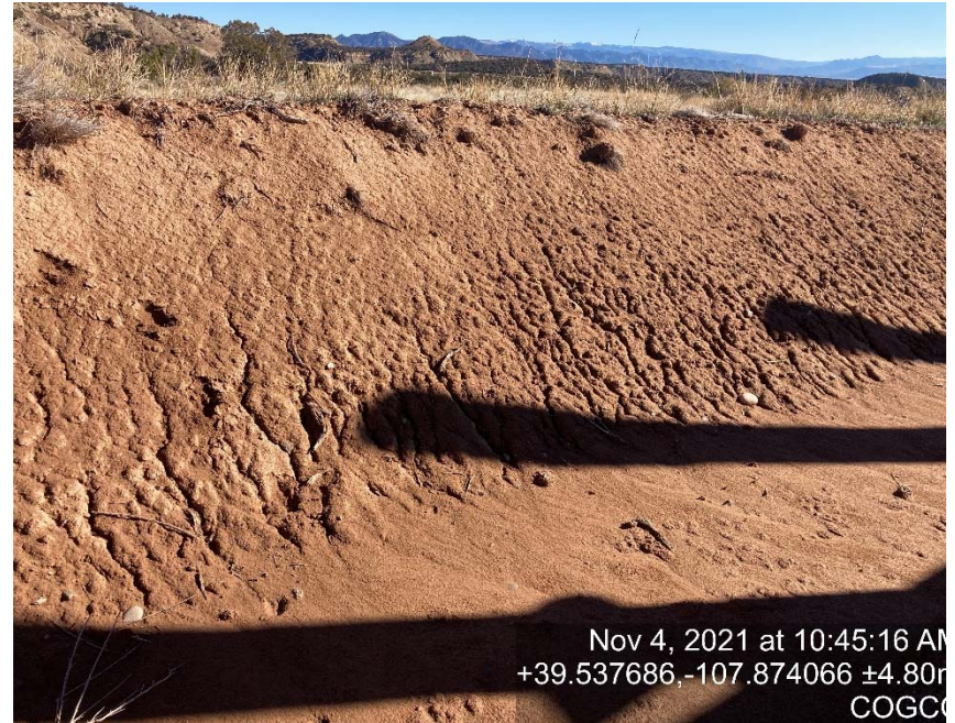
Lack of stabilization/erosion
