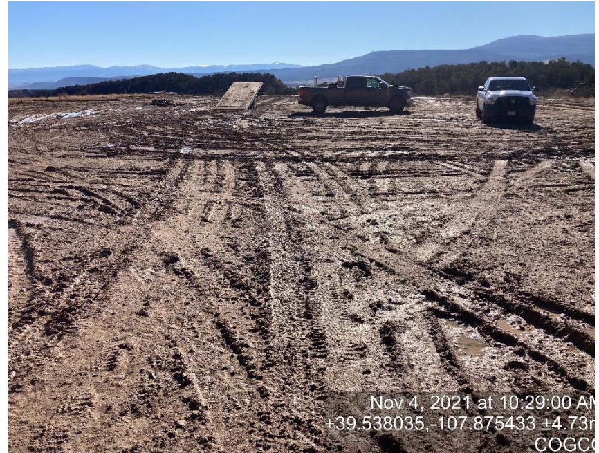
Lack of stabilization/compaction
