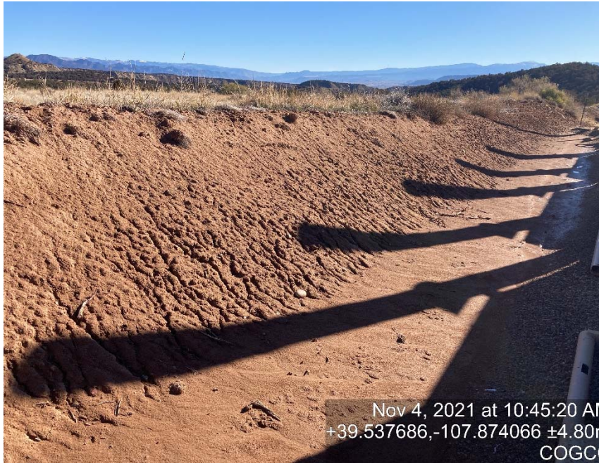
Lack of stabilization/erosion
