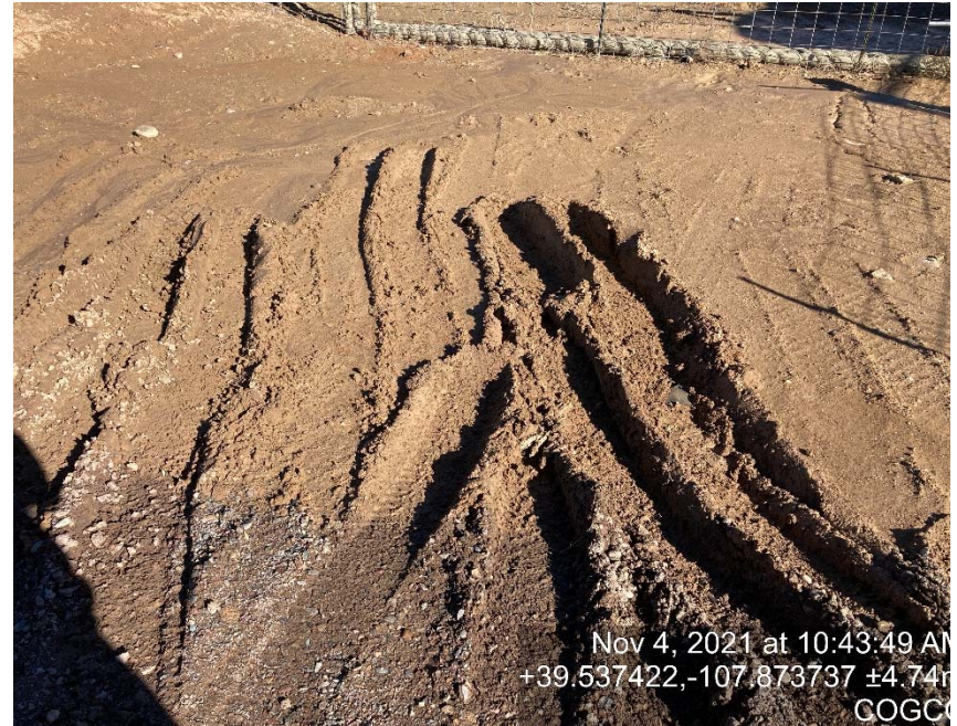
Lack of stabilization/compaction
