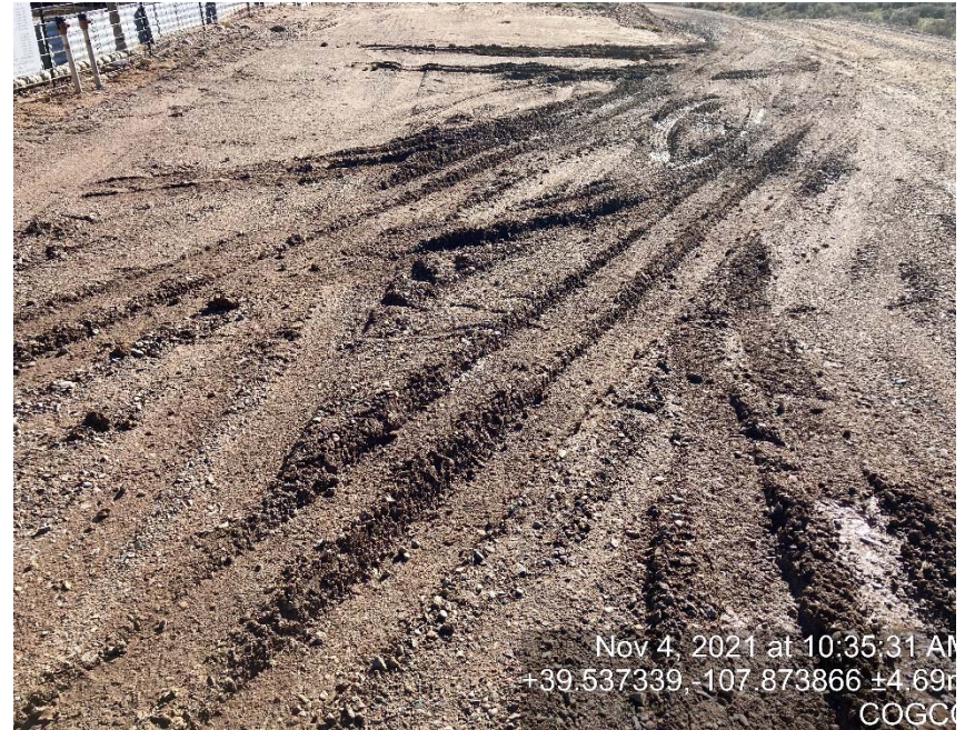
Lack of stabilization/compaction
