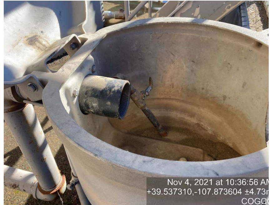
Load out line missing cap/bull plug
